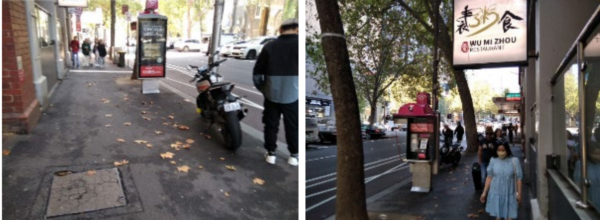
Site Photographs of Cabinet 57 Location, 28 March 2023 [Source: Council Officers]
