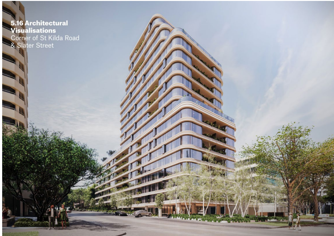
Figure 4 - Render of proposal as viewed from the intersection of St Kilda Road and Slater Street. Source: Permit applicant
