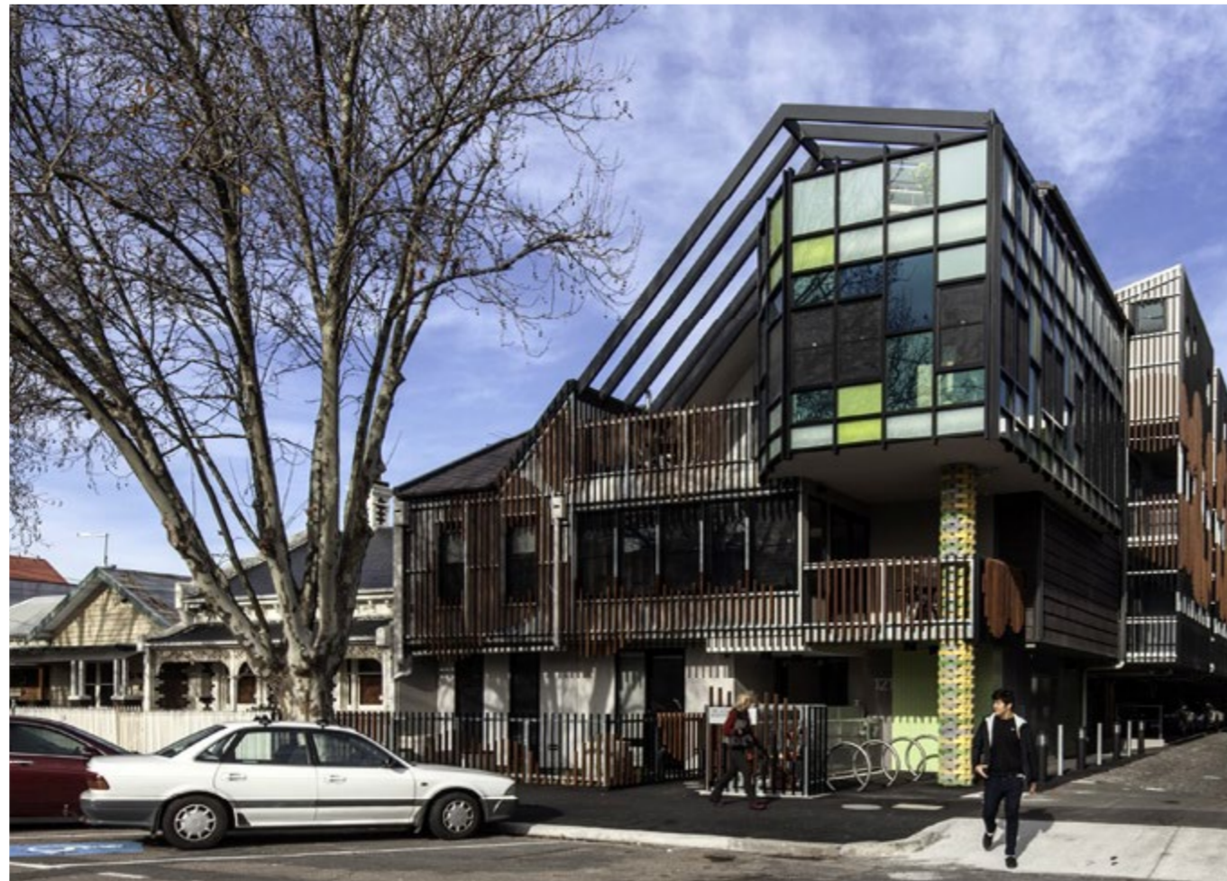
Housing First's affordable housing in Kymes Place, Port Melbourne
