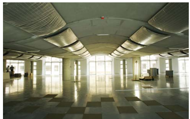
Figure 3: Natural light penetration during construction.
