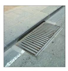
The sawn bluestone overflow kerb is used in combination with side entry pits throughout the municipality.
