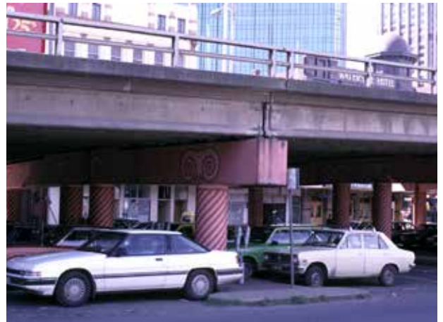
The Flinders Street overpass of King Street, built as part of the Kingsway project, is removed in 2005. The aim is to revitalize the western end of Flinders Street and to enable redevelopment of the car park on the old Fish Market site. [Ron Jones, City of Melbourne]
