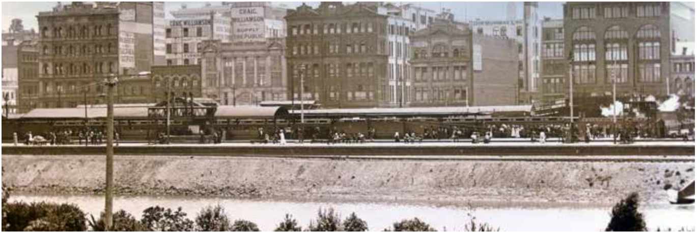
The reconstruction of the river and development of rail stations and yards creates engineered waterway and landscape with little resemblance to the old Birrarung. [John Henry Harvey, State Library of Victoria]
