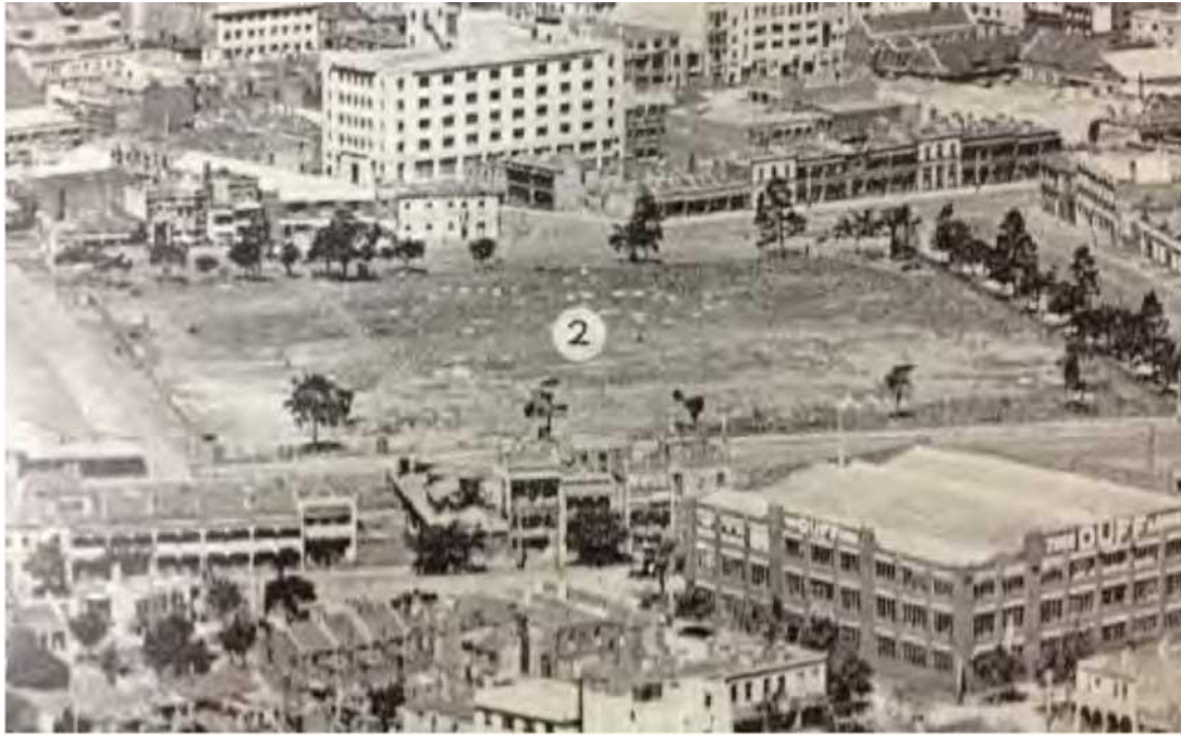
Figure 8 Aerial view of the Old Melbourne Cemetery showing the cleared site, 1928 Source: National Heritage List Assessment: Queen Victoria Market
