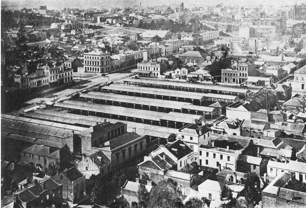
Figure 25 The open sheds of the first Eastern Market, 1873 Source: State Library of Victoria Picture Collection
