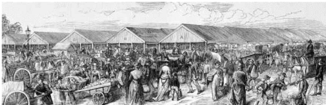
Figure 5 The Queen Street elevations of A to E sheds at the QVM, 1878 Source: State Library of Victoria
