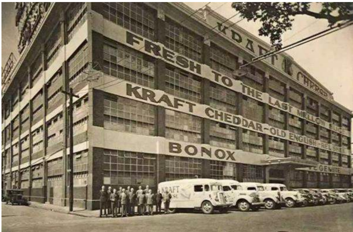
Figure 33 Kraft Factory Southbank (State Library of Victoria)
