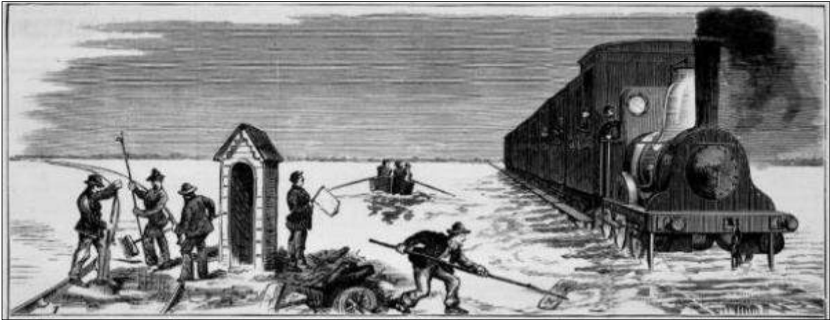
Figure 24 Floods along the Port Melbourne line 66
