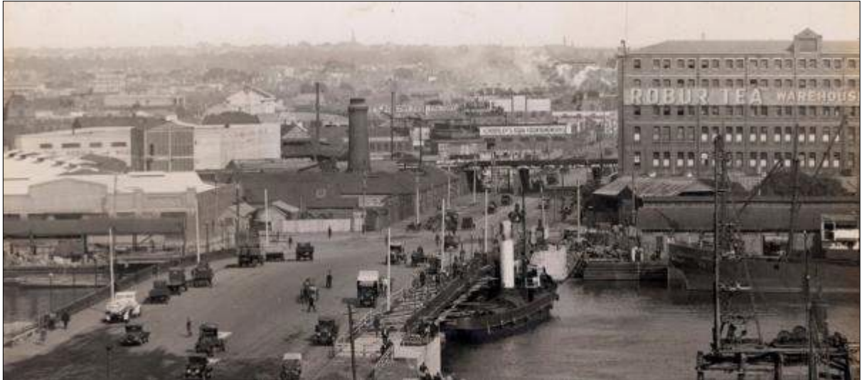
Figure 20 Spencer Street Bridge c.1928 shortly after its completion, showing the densely-developed industrial area, State Library of Victoria H2001.308/3064
