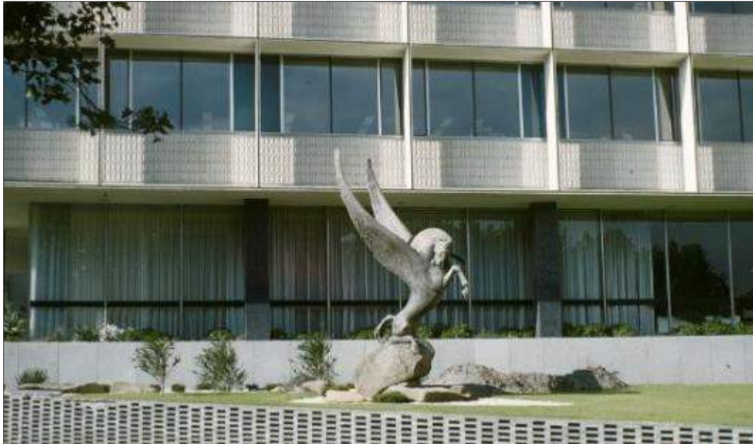
Figure 34 Ewers' Pegasus station and Vacuum Oil building (State Library of Victoria, H91.244/403)
