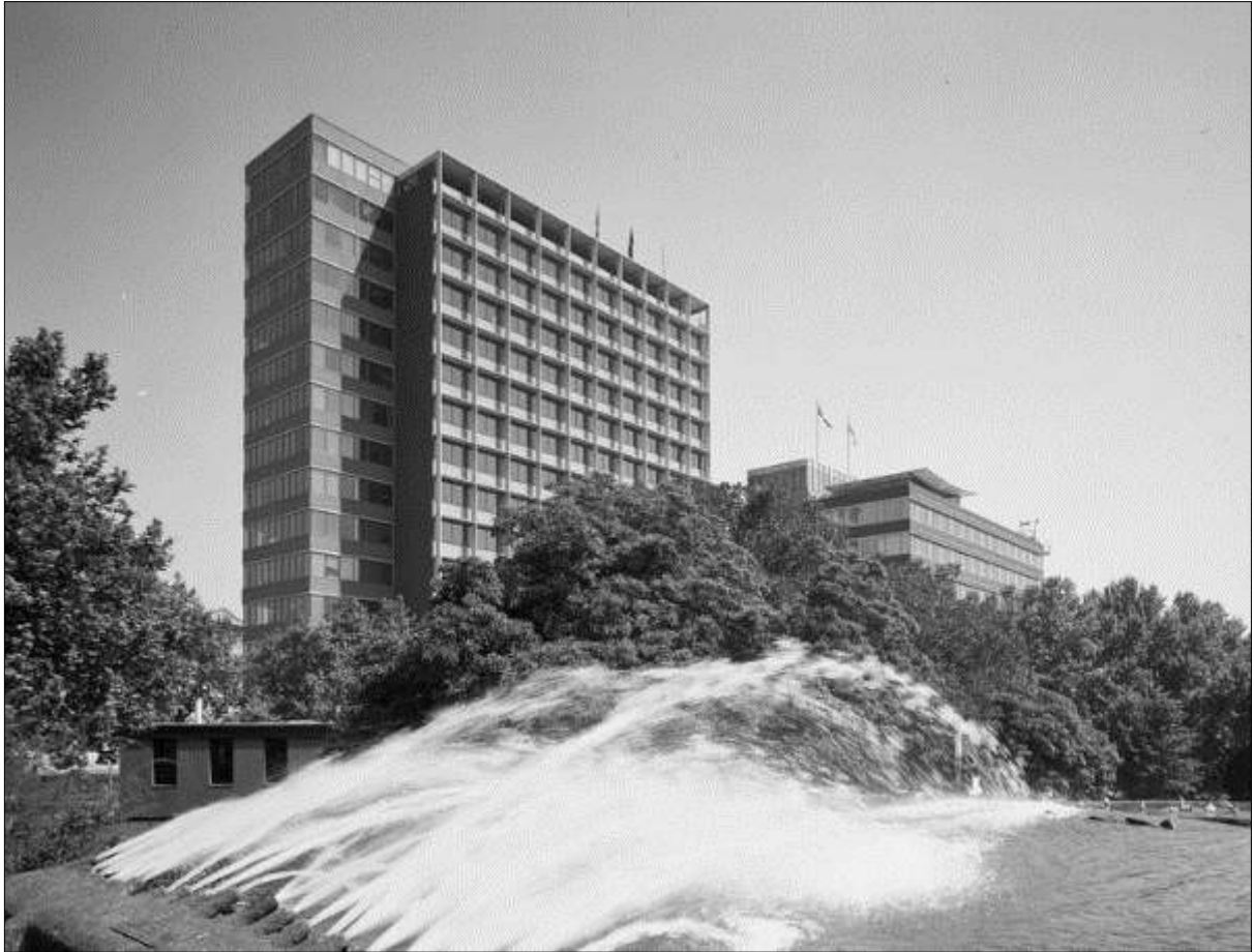
Figure 41 Mobil Oil and APM buildings, South Melbourne, with the Southgate fountain in Snowden Gardens in the foreground (Mark Strizic, 1972, State Library of Victoria H2011.55/1869)
