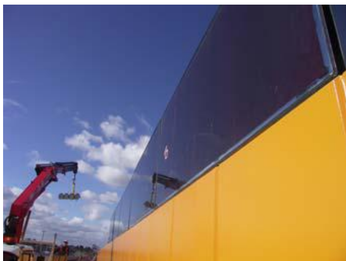
Figure 6: PV noise wall on the Tullamarine Freeway at the Calder Interchange, adjacent to Essendon Airport, Melbourne. Source (TCI, 2009)
