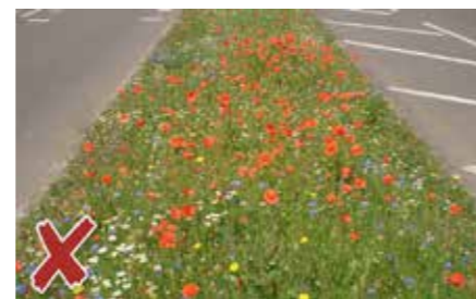
Planted median with insufficient offsets for access
