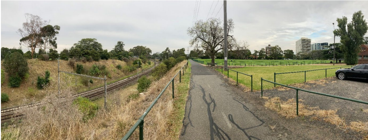
Photo 2 Upfield rail line in a deep cutting before near Poplar Oval, looking northeast
