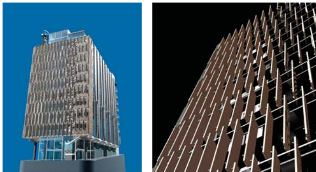
Figure 6: Concept images of CH 2 west façade showing movable wooden louvers for shielding against heat gains from low western sun – an expression of bioclimatic architectural language.
