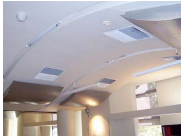
Figure 14. Prototype full scale of the office spaces with precast concrete ceiling-floor system
