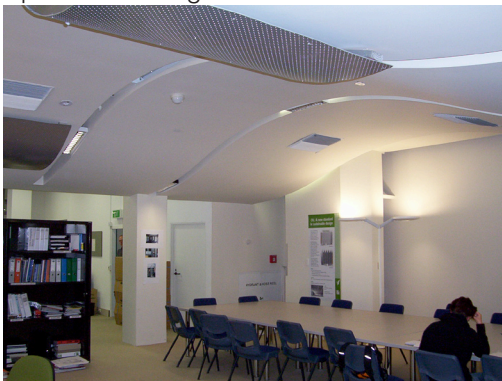
Figure 2. Testing different fixtures in the wave ceiling prototype
