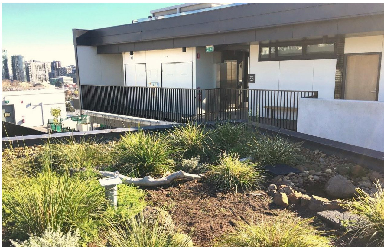
Biodiversity green roof located on Hawke and King Apartments, West Melbourne. This green roof was planted with Lomandra longifolia , Poa labillardieri and Themedia triandra in early 2018. It includes two perching logs, eight large volcanic stones and a small ephemeral pond, for shelter and a semi-reliable water source. Photo: Ben Nicholson, The Urban Greener.
