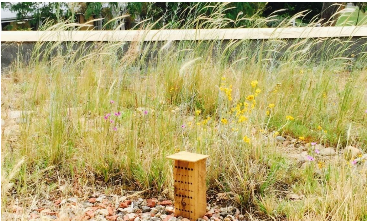
A patch of substrate made from broken bricks and an insect hotel on the Burnley Biodiversity Green Roof. Photo: Nicholas Williams.
