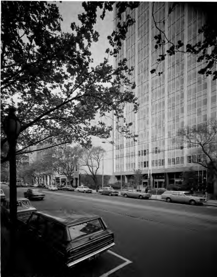
Figure 3. Conzinc-Rio Tinto Building at 95 Collins Street, 1970 (State Library of Victoria, H2011.55/1479)
