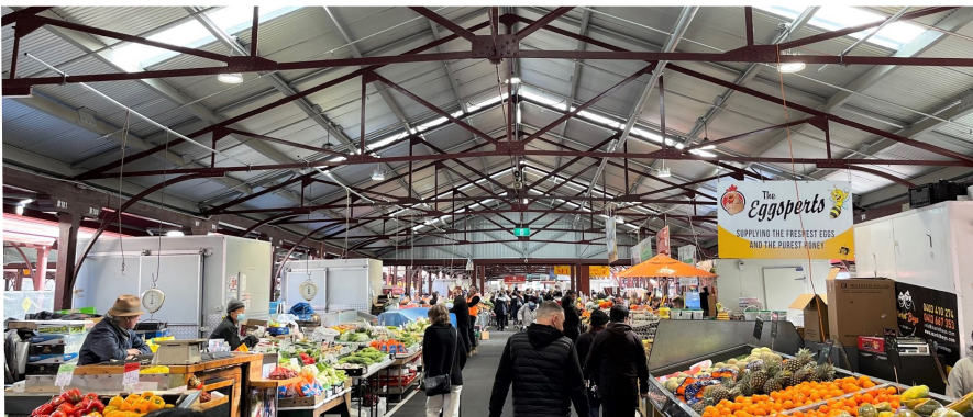
Photo: Recently restored Shed B
