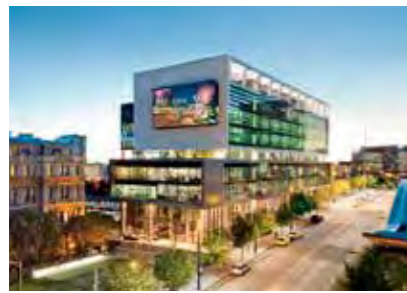
Media House and Collins Street Bridge, Docklands
