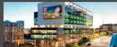
Development over road and rail infrastructure – Media House and Collins Street Bridge, Docklands
