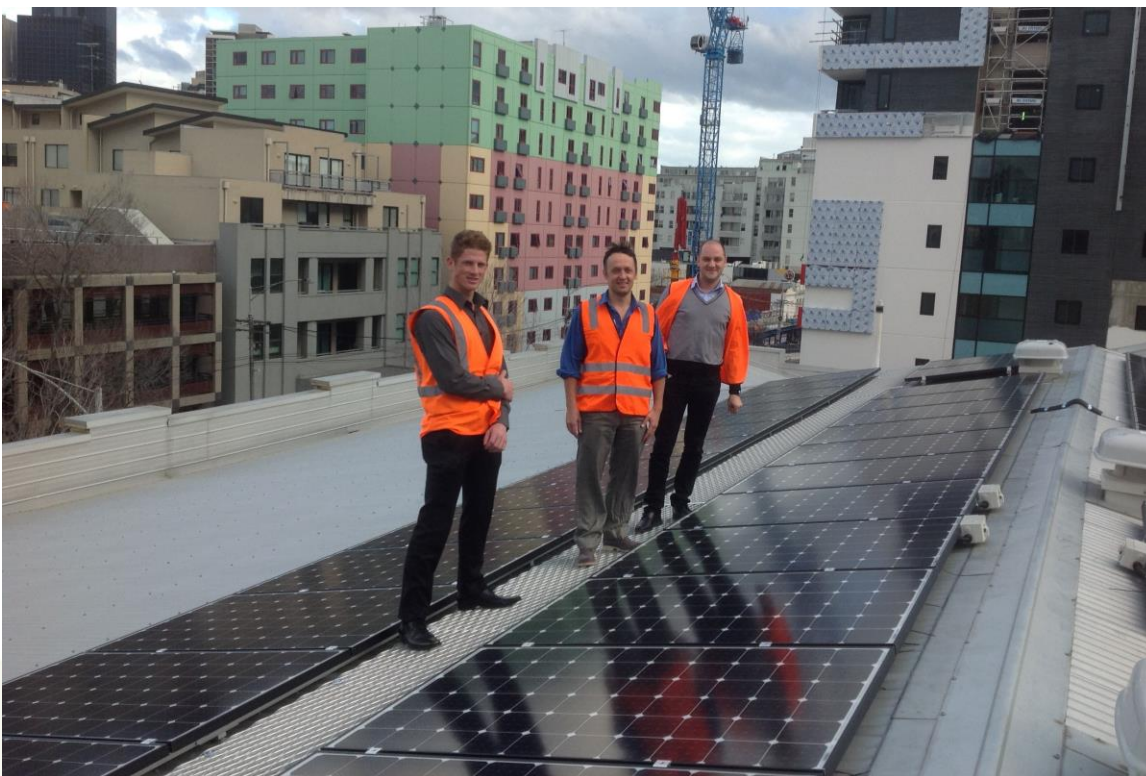
Harry Troedel (pictured middle) inspects the new solar installation system.
