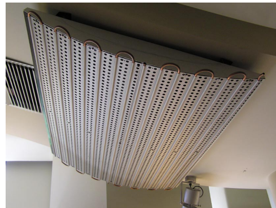
Figure 10. Chilled ceiling prototype
