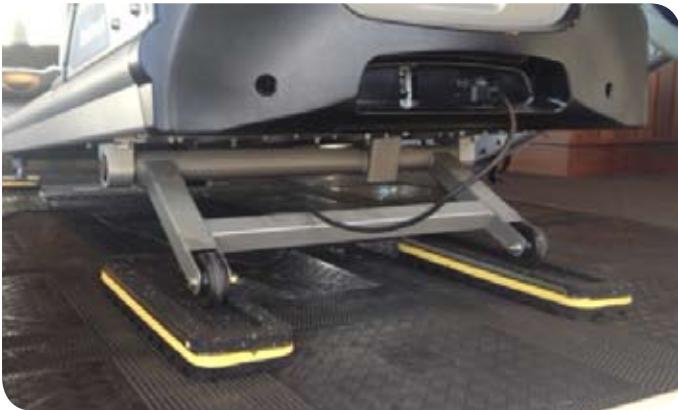
Acoustic isolation of a running machine to minimise noise transfer (FMV)
