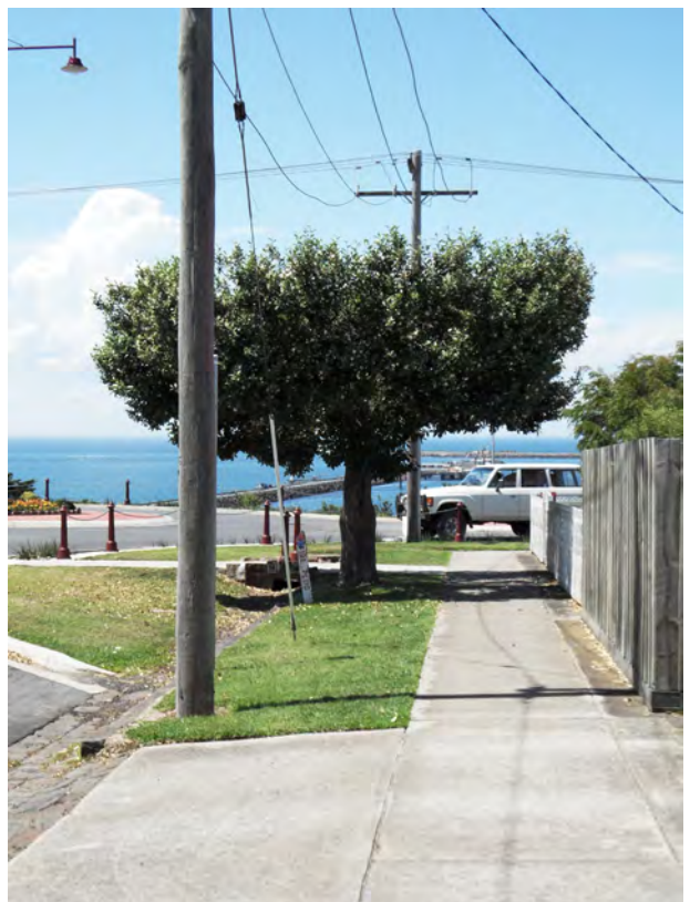
Trees pruned heavily around power lines
