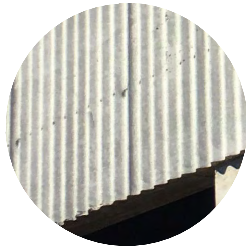
CON1 - PRECAST CONCRETE WALL PANEL
