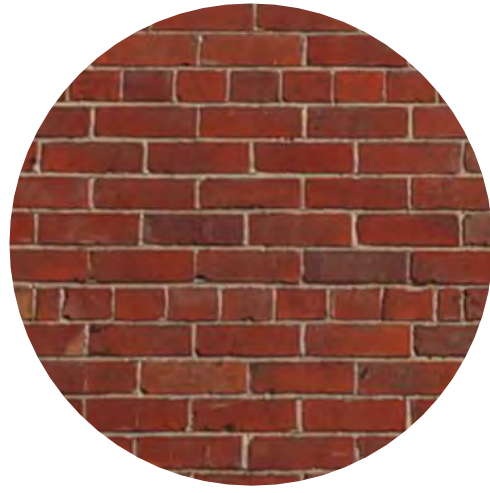
EXISTING CHURCH BRICKWORK
