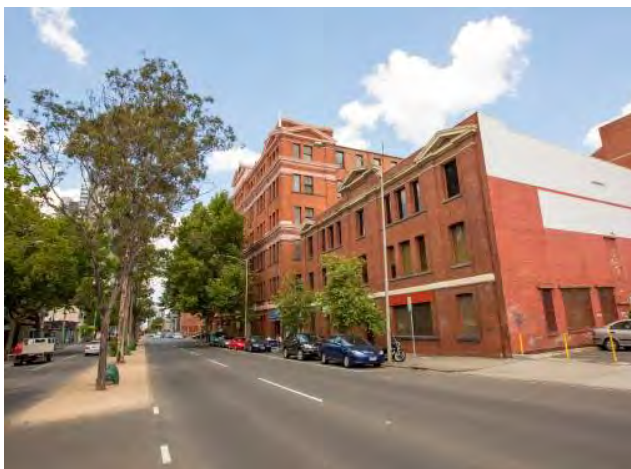
Figure 17 Sands & McDougall buildings
