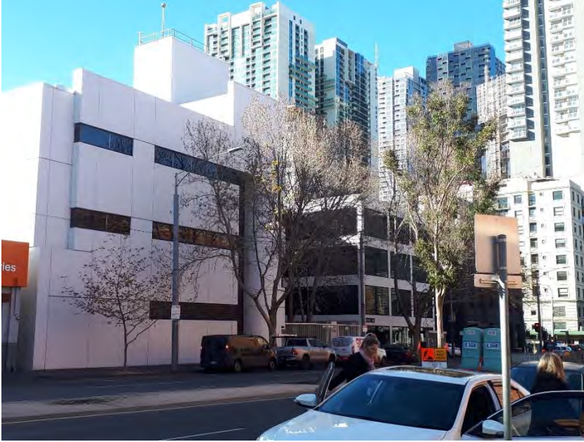
Figure 19 Current development on 328-348 Spencer Street
