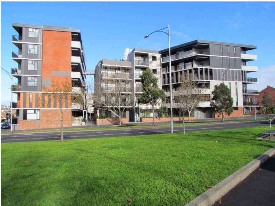
Figure 4: New 6 storey mixed use to west of Miami (King Street frontage)
