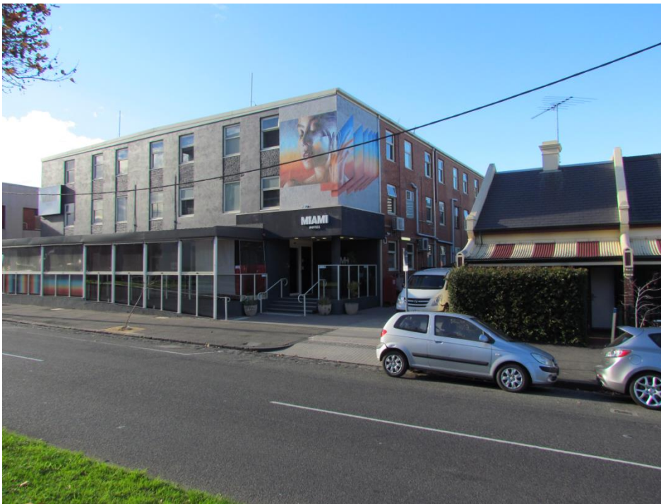
Figure 2: Miami Hotel (existing frontage to Hawke Street)
