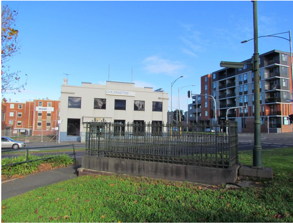
Figure 5: Miami Hotel, Goldsmiths building and new 6 storey mixed-use (from north)
