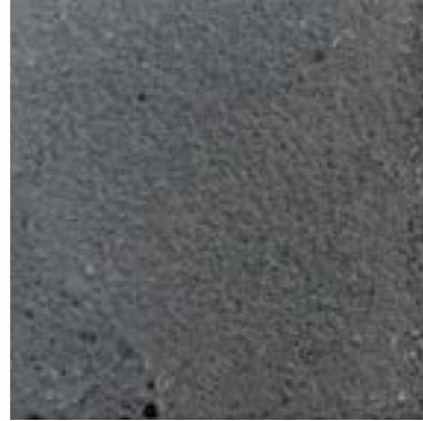
Grit blasted feature pavers
