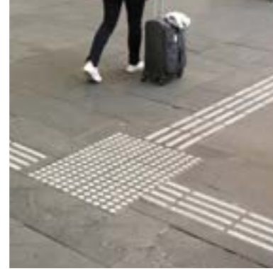
Hazard and directional tactile indicators
