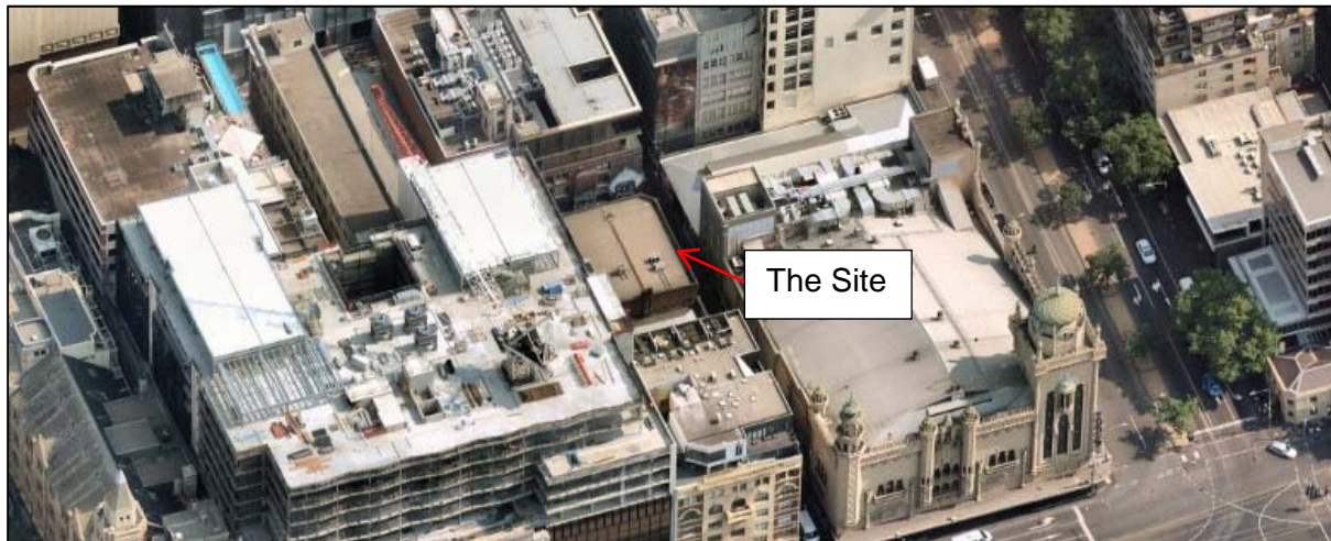
Figure 3: Aerial view of the Site (NearMap image dated 17/12/2019)
