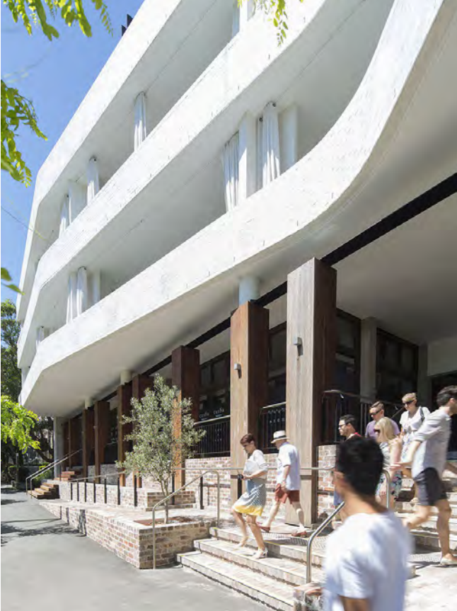
Image 11: The design successfully addresses the transition in floor levels by incorporating a ramp, stairs, seating and planting. The double height ground floor further improves street activation and daylighting to the tenancies.
