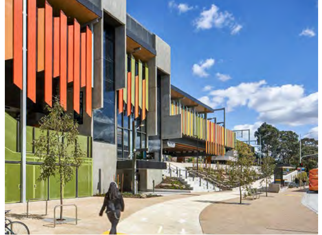
Image 23: The new Rosanna Station as part of the Victorian Government's Level Crossing Removal Project.
