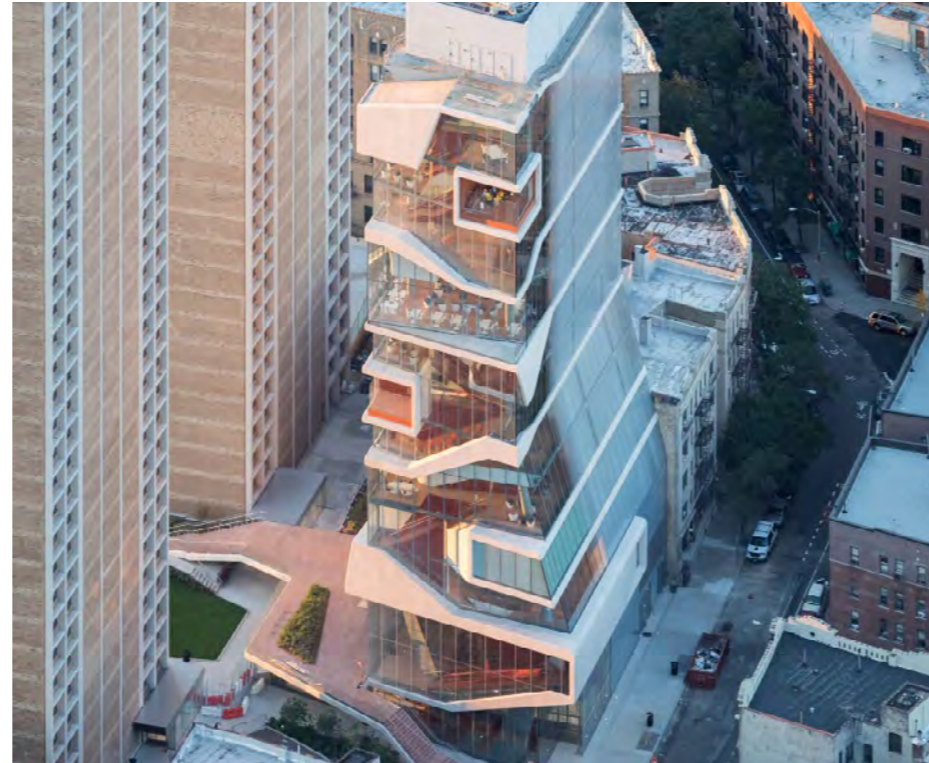
Columbia University's Vagelos Education Centre is a 14 level vertical school for the University's Medical School. It emphasises the importance of informal break-out, informal learning space by expressing a continuous public stair called the "Study Cascade" at the facade.
