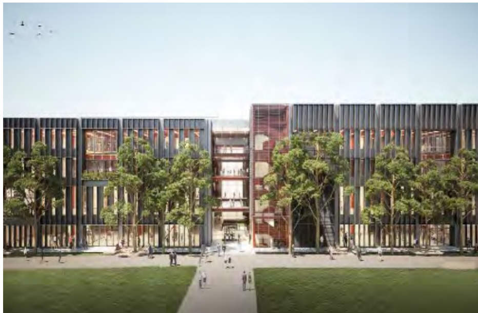
Monash University's upcoming Technology Education building is a long, 5 level structure that focuses on long spans to allow for very large, highly flexible, column free classroom/testing spaces.
