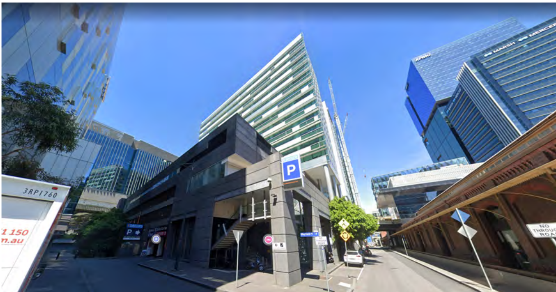
Figure 6: Building to be demolished at corner of Mayfield Place and Aurora Lane (Google Street View)
