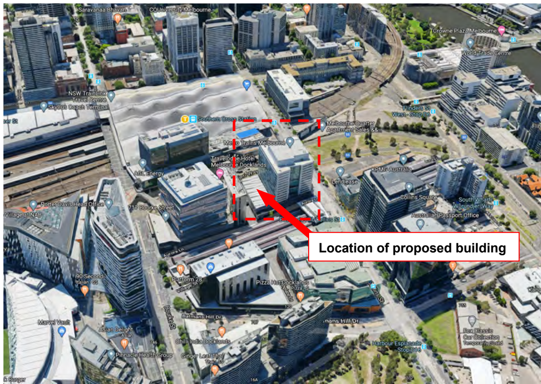
Figure 4: 3D aerial of subject site's immediate built form context (Google Maps)
