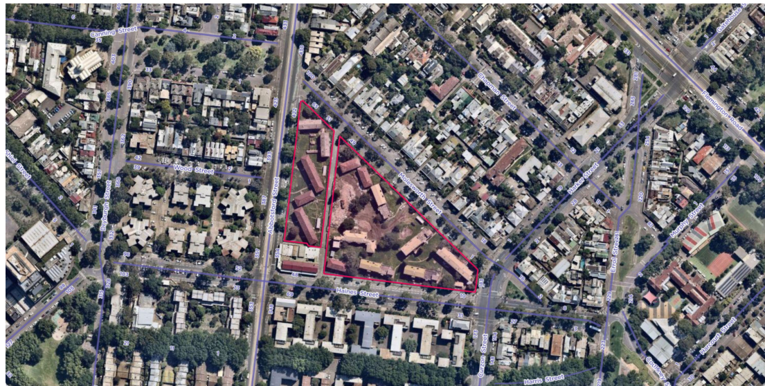
Figure 2: Aerial of subject site and surrounds (NearMap 17 February 2020)
