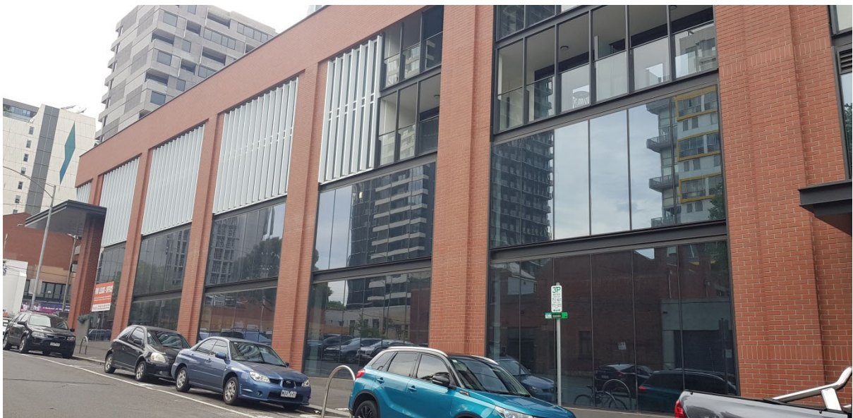
Figure 2: Site Photograph (10 November 2020)
