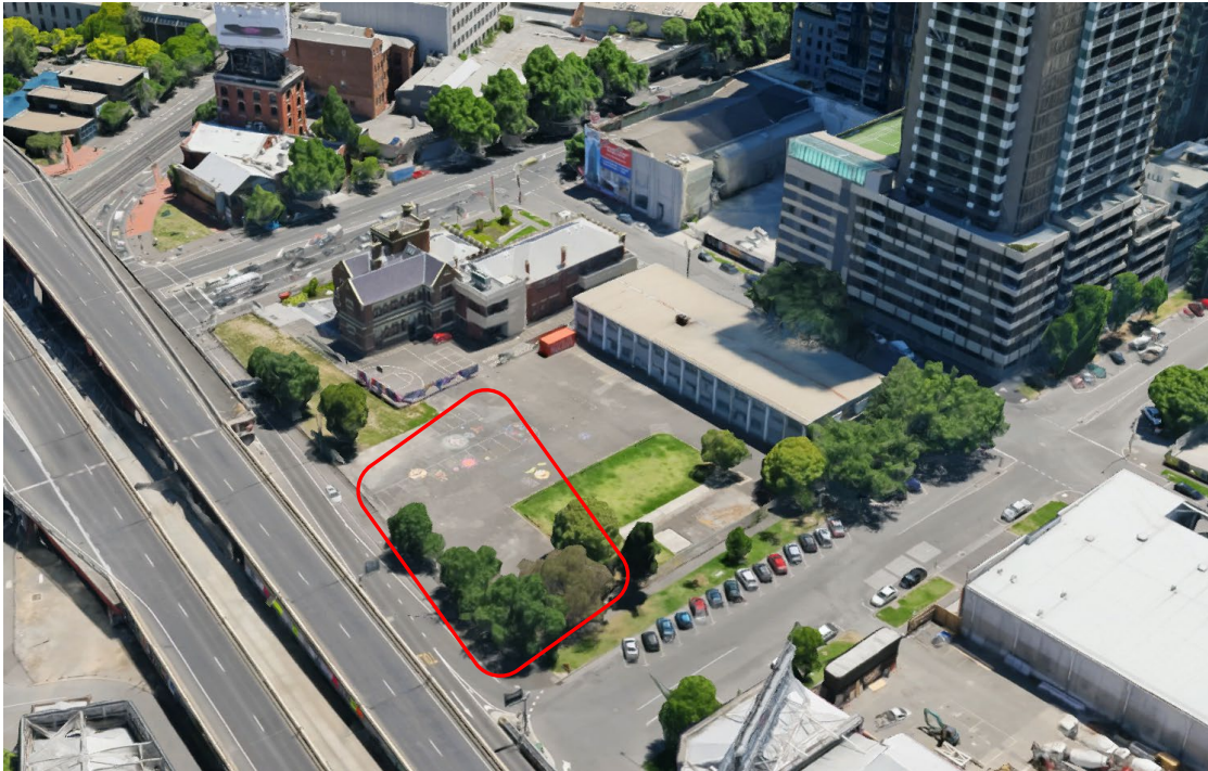
4. 3D aerial of subject site's immediate built form context (Google Maps). *Note the building along Balston Street has been removed and the works to Boyd Park have commenced.
