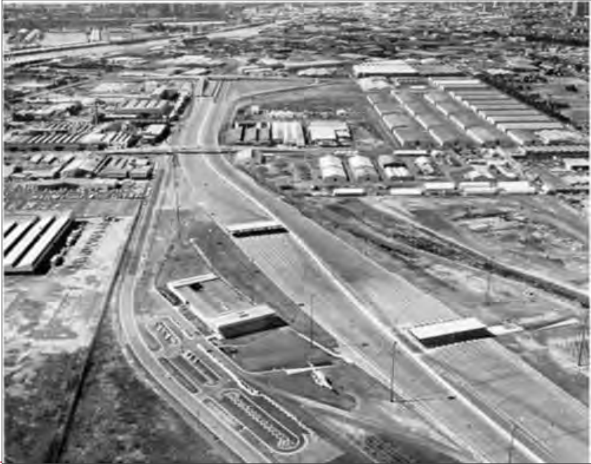
Figure 37—West Gate Bridge toll plaza looking east just prior to opening (Museum Victoria)
