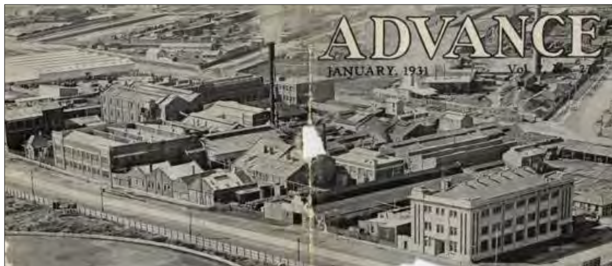
Figure 16—Kitchen & Sons factory, from company brochure
