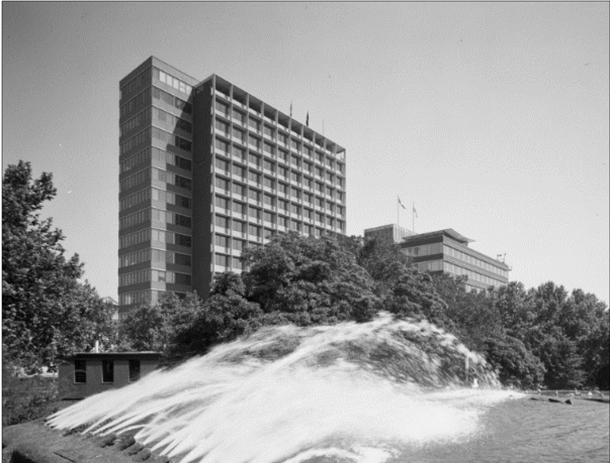
Figure 41 Mobil Oil and APM buildings, South Melbourne, with the Southgate fountain in Snowden Gardens in the foreground (Mark Strizic, 1972, State Library of Victoria H2011.55/1869)
