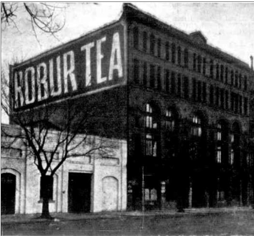
Figure 13 107-127 Queens Bridge Hotel as shown in 1907 publication
