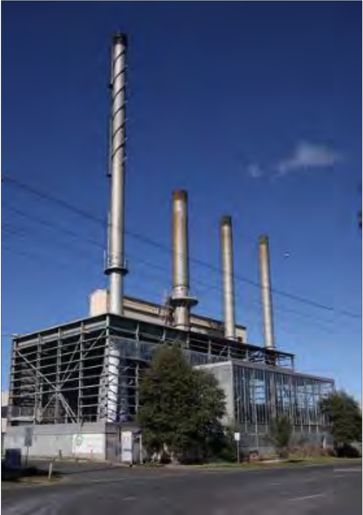
Figure 62— Demolished Holden boiler house (Marcus Wong)
