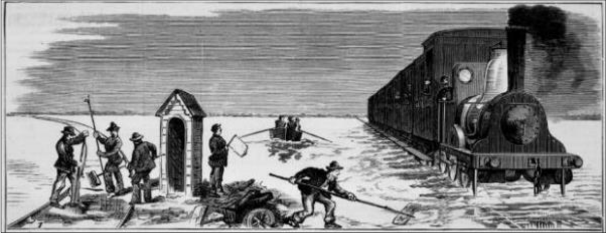
Figure 24 Floods along the Port Melbourne line 102
