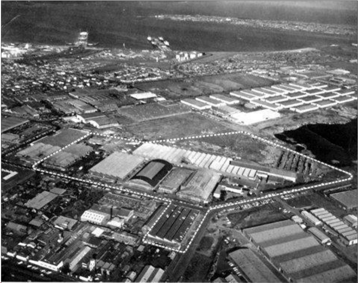
Figure 65—AMI Factory, Port Melbourne, 1960s 147
