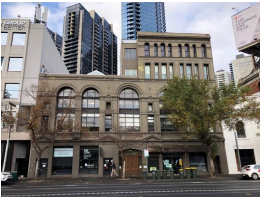
Figure 14 Current condition of 107-127 Queens Bridge Hotel
