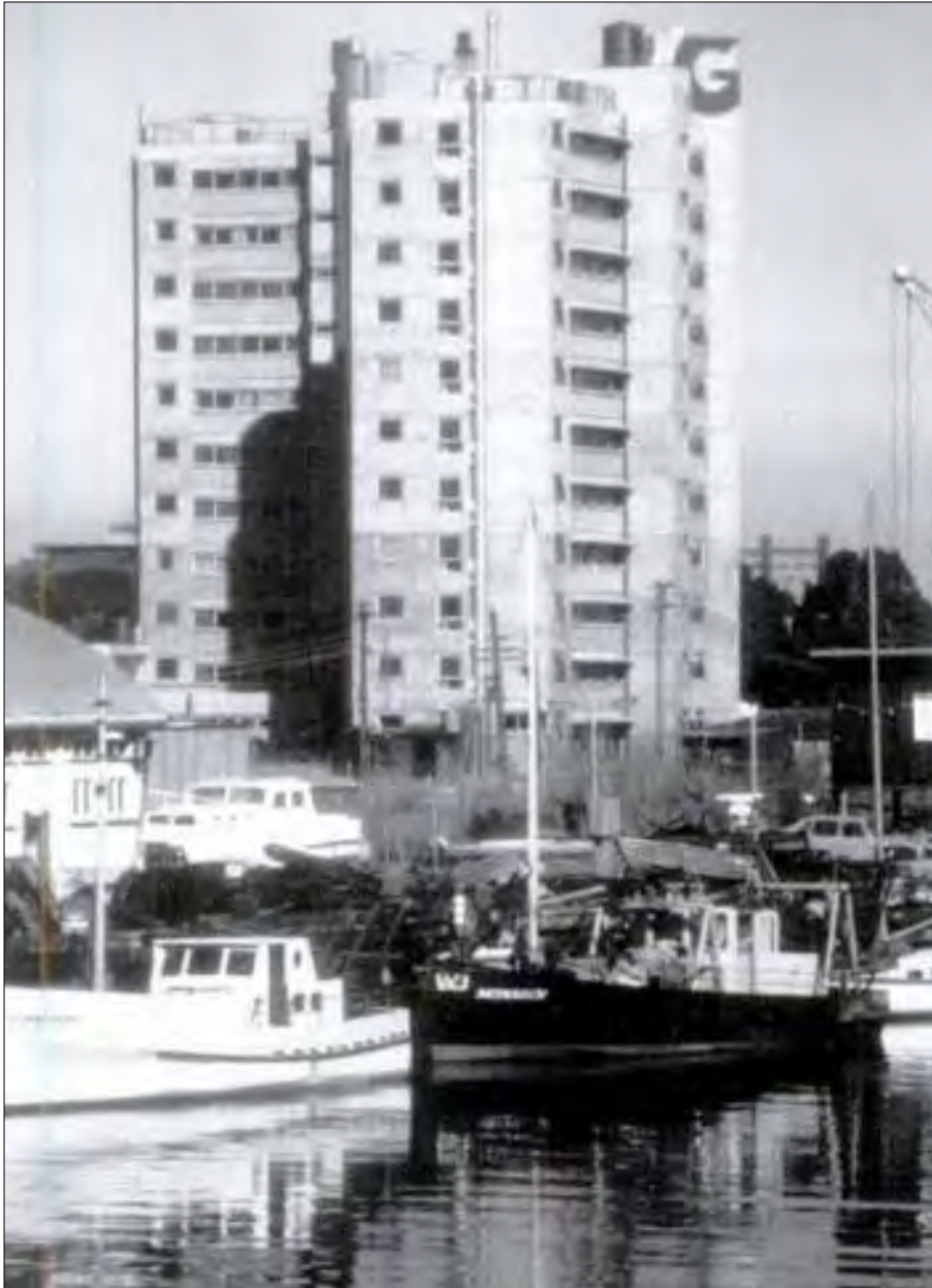
Figure 26 New Gordon House
