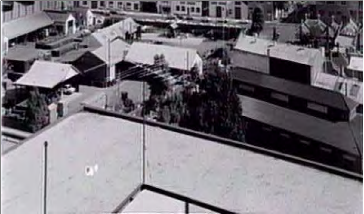
Figure 28 Looking over Dorcas Street and Lanes Motors to the small factories and warehouses of South Melbourne (State Library of Victoria)
