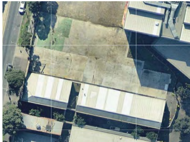
(Shows the retention of the southern roof form and part of the façade of the middle roof form, source: Nearmap)
