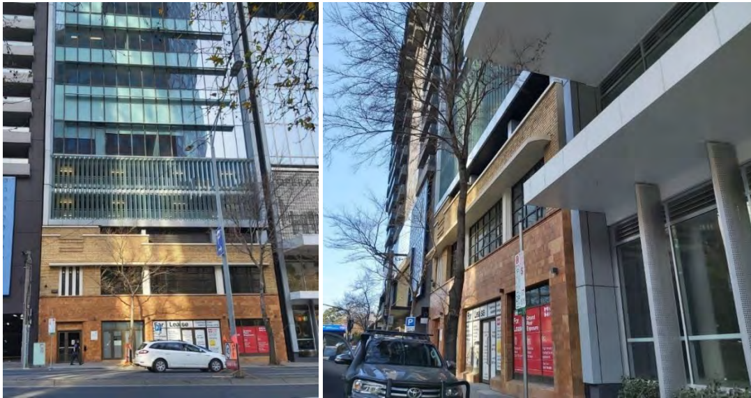
Figure 6 35-41 City Road existing conditions
