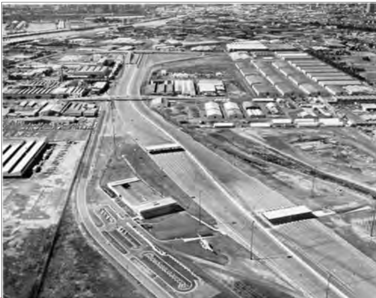
Figure 37—West Gate Bridge toll plaza looking east just prior to opening (Museum Victoria)
