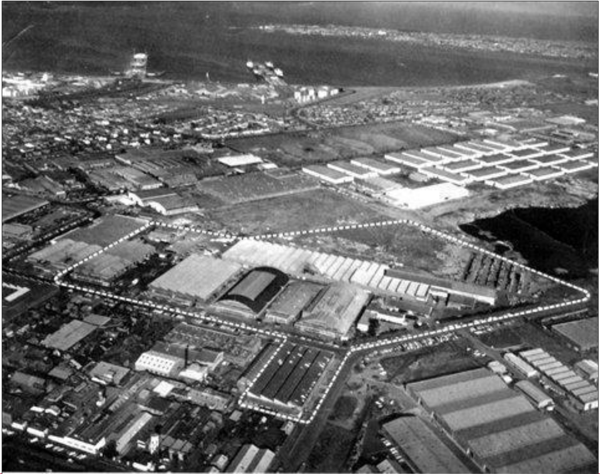
Figure 65—AMI Factory, Port Melbourne, 1960s 147
