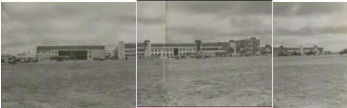
Figure 46—CAC from the south showing camouflage-painted buildings 127
