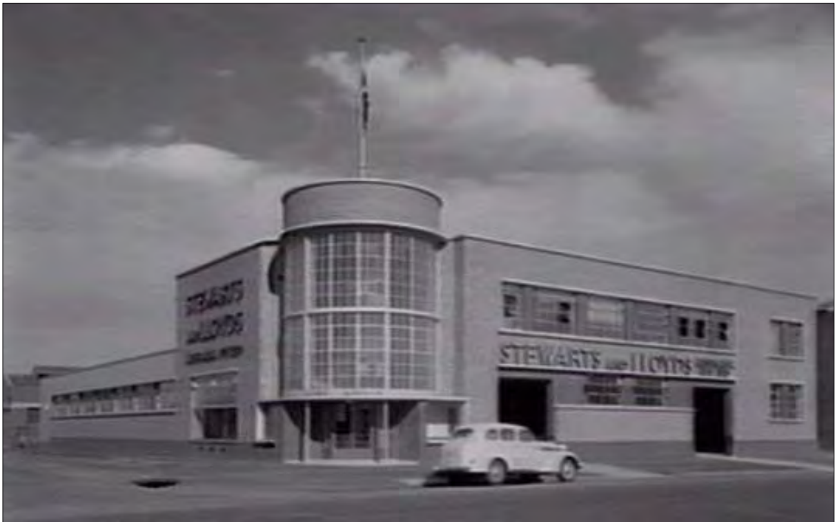
Figure 32 Stewarts & Lloyds head office, City Road (Museum Victoria)
