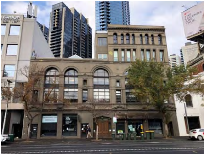
Figure 14 Current condition of 107-127 Queens Bridge Hotel
