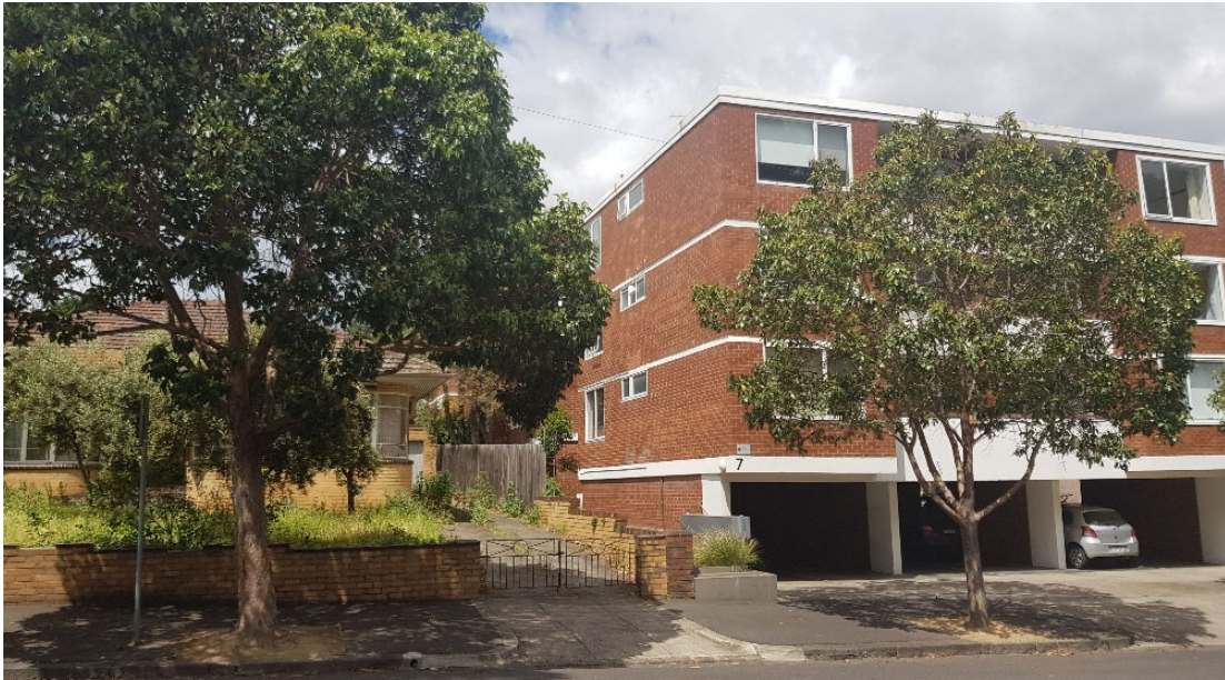
Figure 3. 7 Curran Street adjoining the subject site (Source: Site visit)
