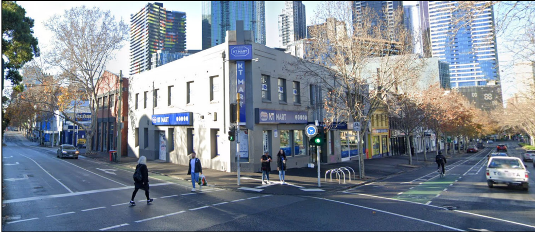
Figure 4: Subject site from corner of Elizabeth Street and Queensberry Street (Google Street View)
