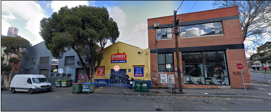
Figure 7: Subject site from Berkeley Street (Google Street View)
