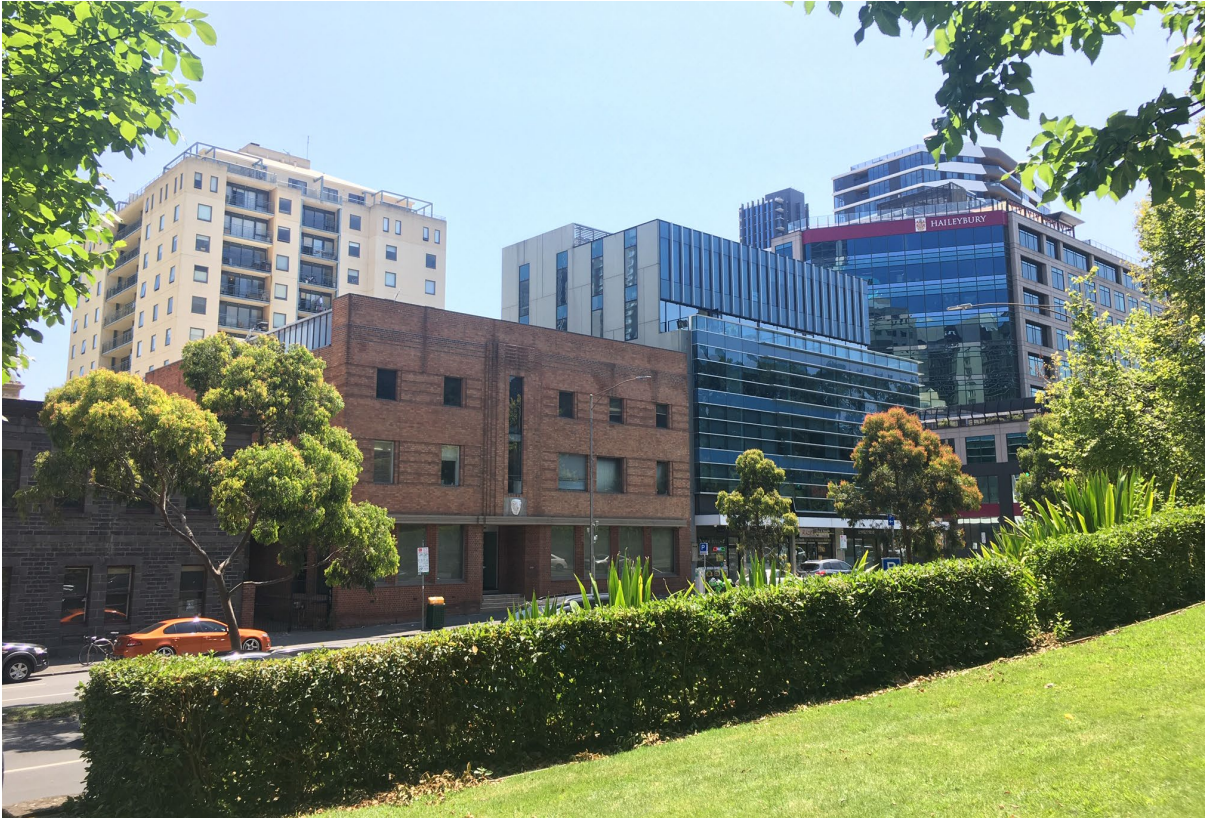
Figure 3 - View of site from Flagstaff Gardens. Taken on 23 January 2020
