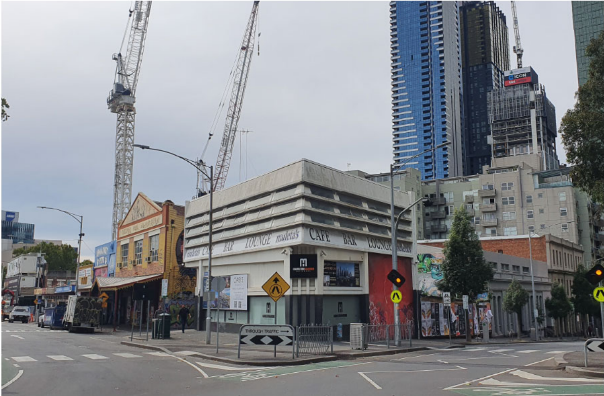
6. The Site – corner Queen Street and Franklin Street (facing north-east): Photograph by BatesSmart Pty Ltd
