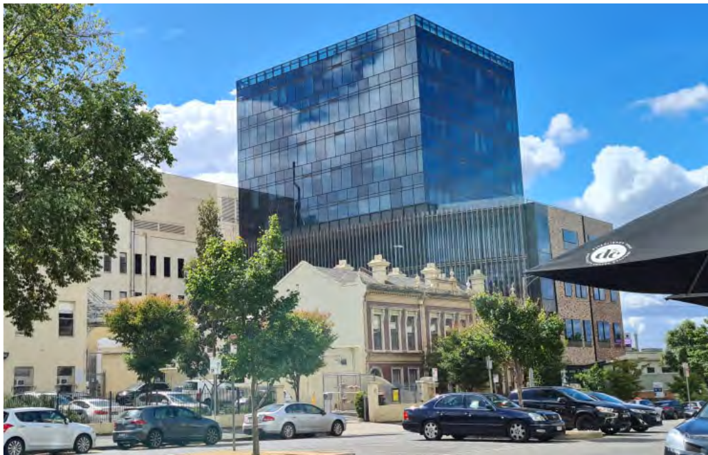
Above: Photograph of Stage 1 viewed from Grey Street
