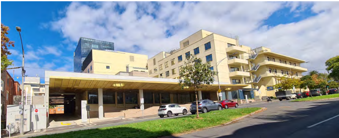
Above: Photograph of Stage 1 viewed from Albert Street and original Freemasons building
