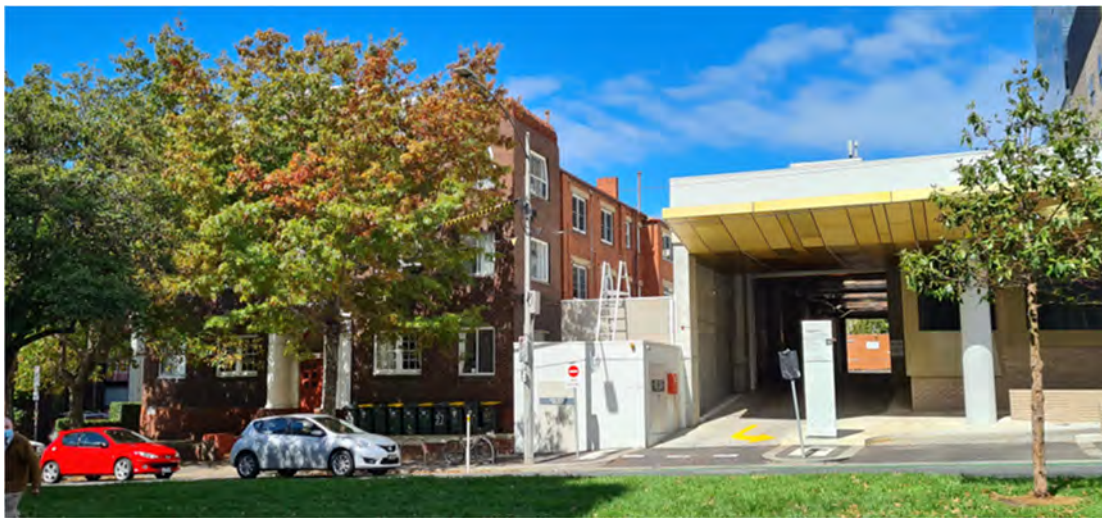
Above: Photograph of 97 Albert Street (left) and Stage 1(right)
