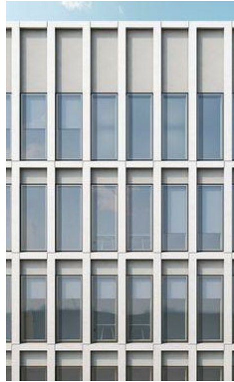
TOWER - A LIGHTWEIGHT EXPRESSION OF THE GRID WHICH OFFSETS ITS HEAVIER PODIUM DESIGN
