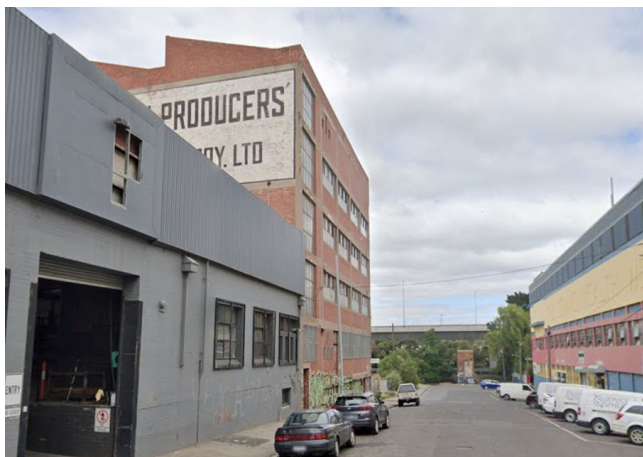
Above: Photograph of signage at 85 Sutton Street, North Melbourne
