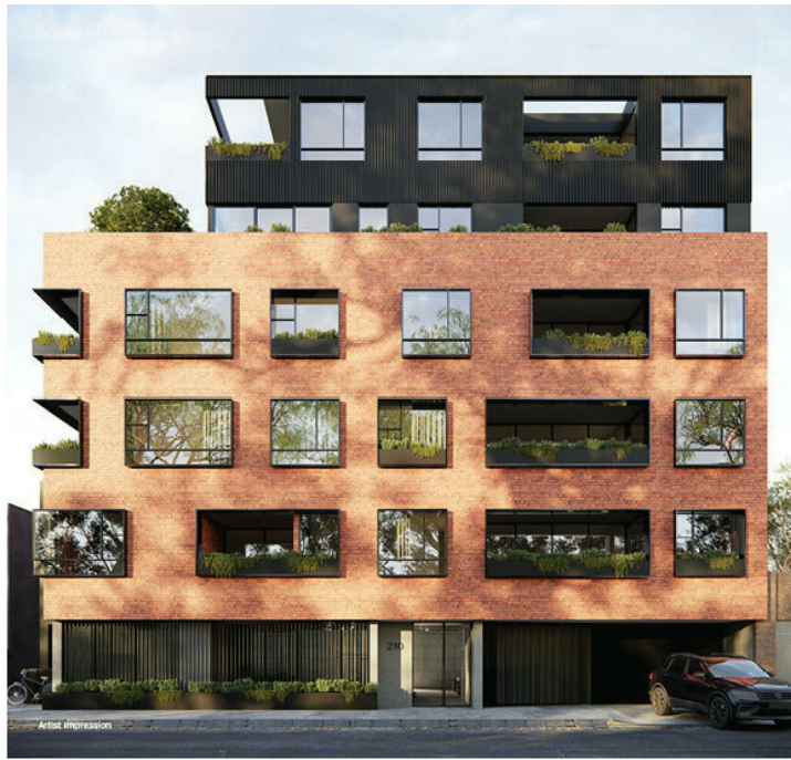
BRICKWORK – CONTINUATION OF MATERIALITY FROM ADJACENT HISTORIC BUILDING IN A CONTEMPORARY FORM.
