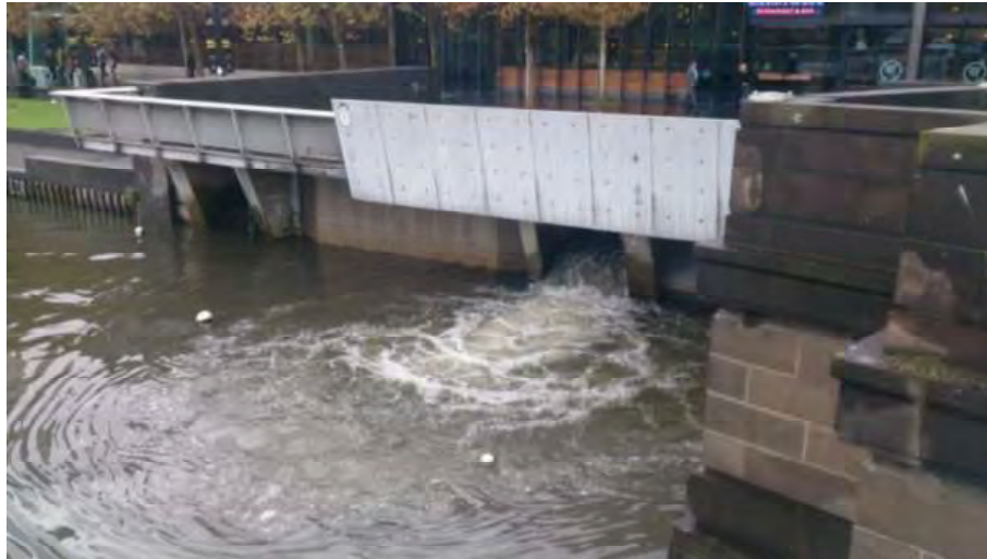
Figure 5-1 Pumped discharge from the Crown Entertainment Precinct
