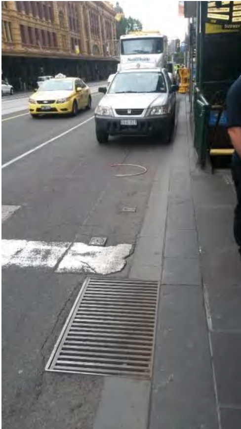
Figure 0-1 Grated kerb pit on Flinders Street, adjacent Degraeves Street Underpass
