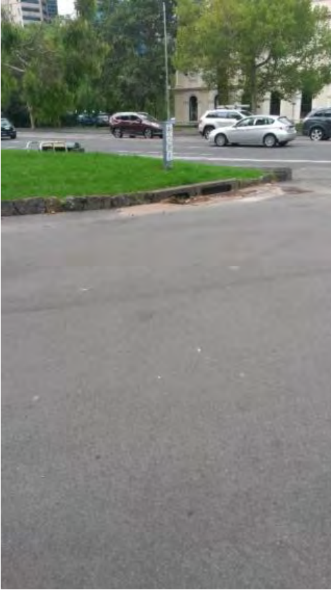
Figure 0-5 Double Side Entry Pits at Carlton Gardens entrance
