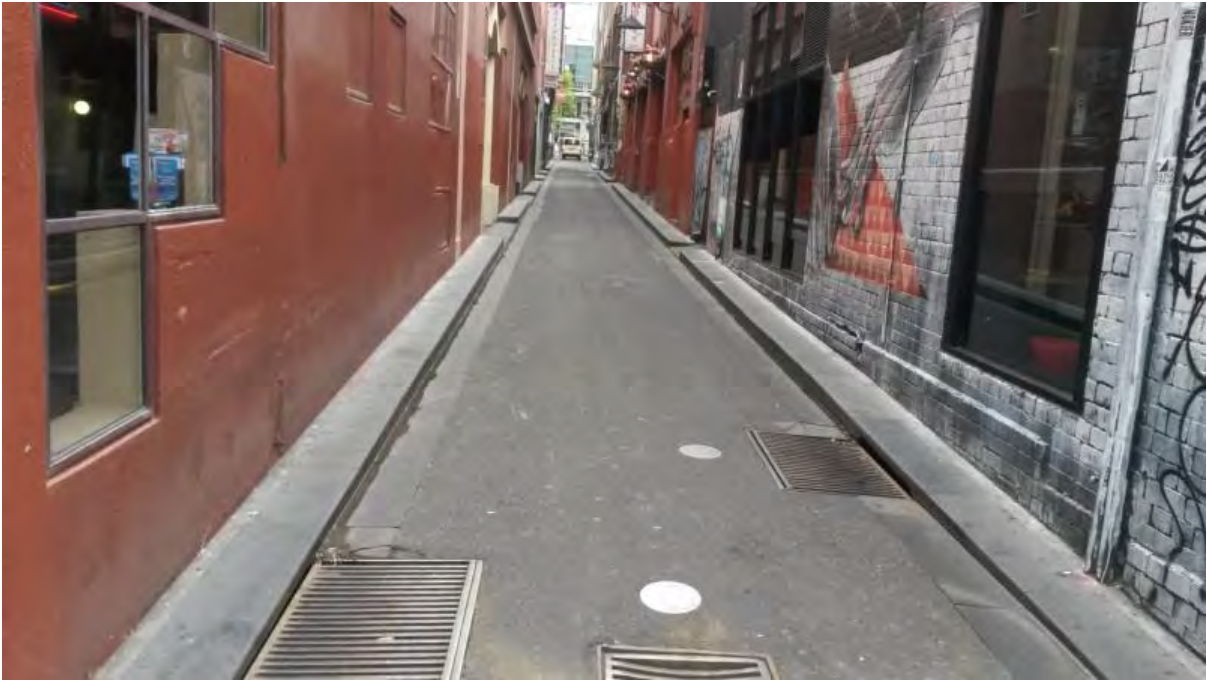
Figure 0-3 Typical grated kerb pits and lane-type pits
