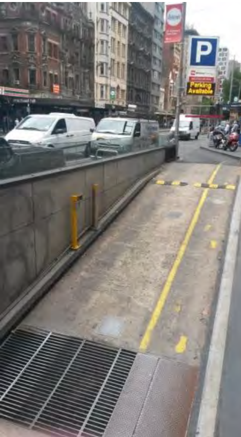
Figure 0-6 Entrance to car park on Elizabeth Street, near Little Collins Street
