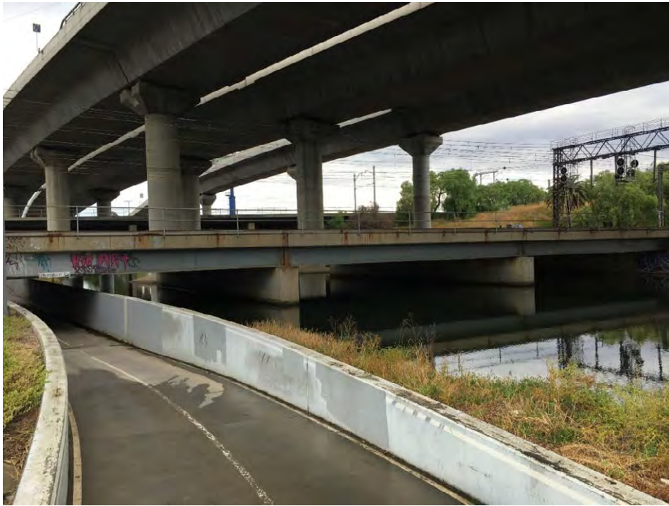
Figure 2.4 Rail bridge downstream of Arden Street (looking downstream)
