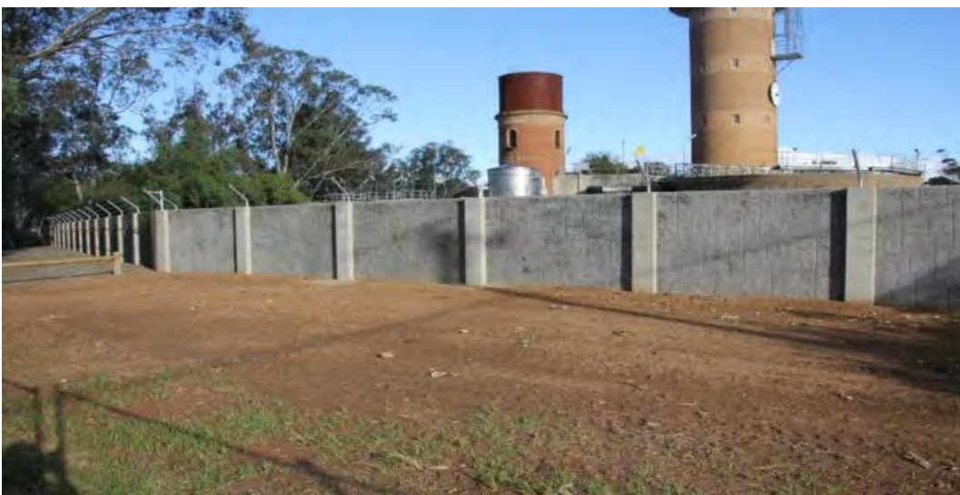
Flood protection levee – Rochester Water Treatment Plant
