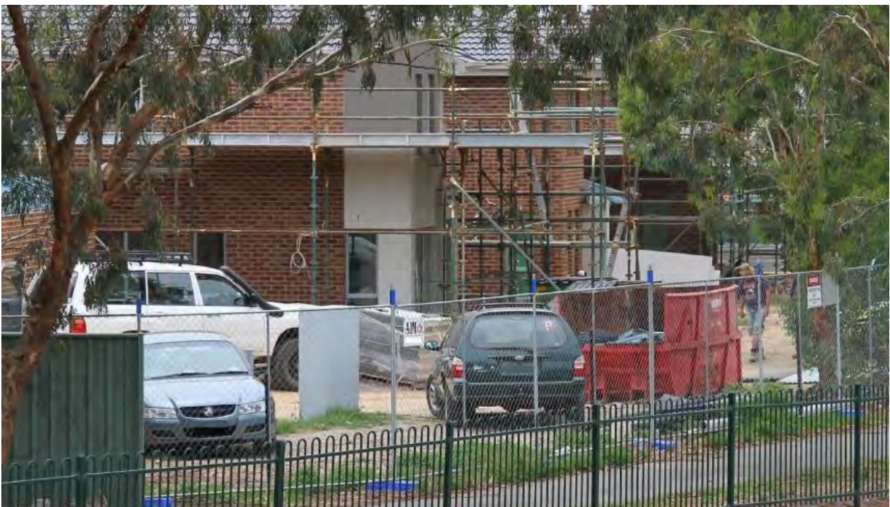
Construction adjacent to a creek in Bendigo
