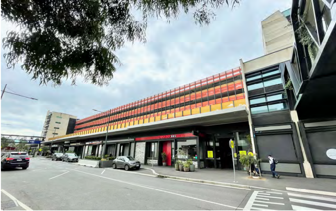
Figure 5 – West elevation of the existing building on the site, taken on 23 March 2021
