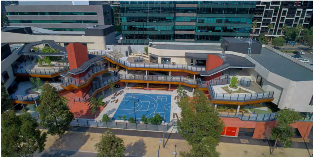
Figure 6 – Docklands Primary School (Source: www.schoolbuildings.vic.gov.au )
