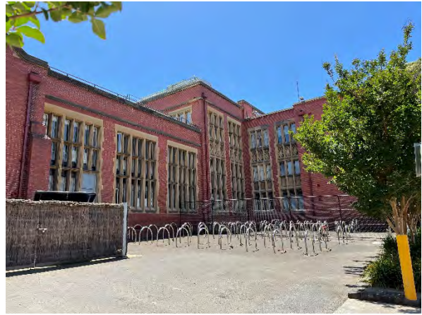
Figure 2 Peter Hall Building (HO820)
