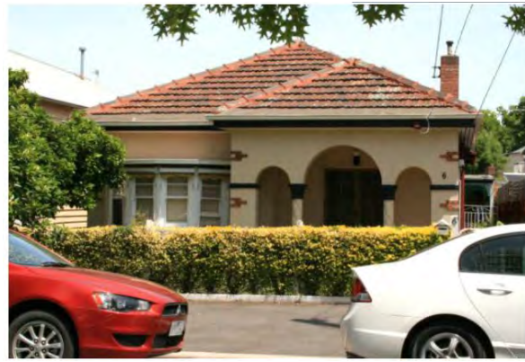
Figure 4 Waddington's houses, 6 Parsons Street, Kensington (HO1167)
