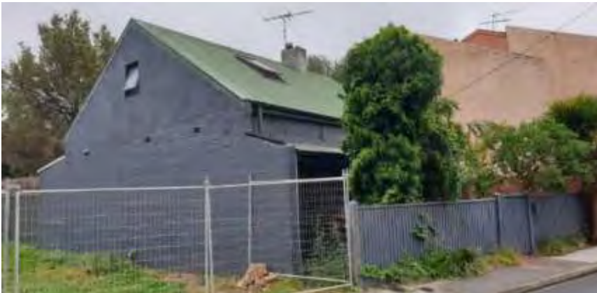
Figure 5 Western wall of dwelling at 99 Buncle Street, North Melbourne
