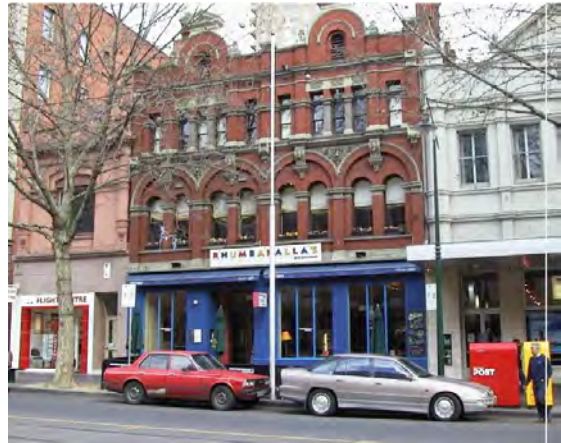
Figure 2 23-29 Bourke Street, Melbourne
