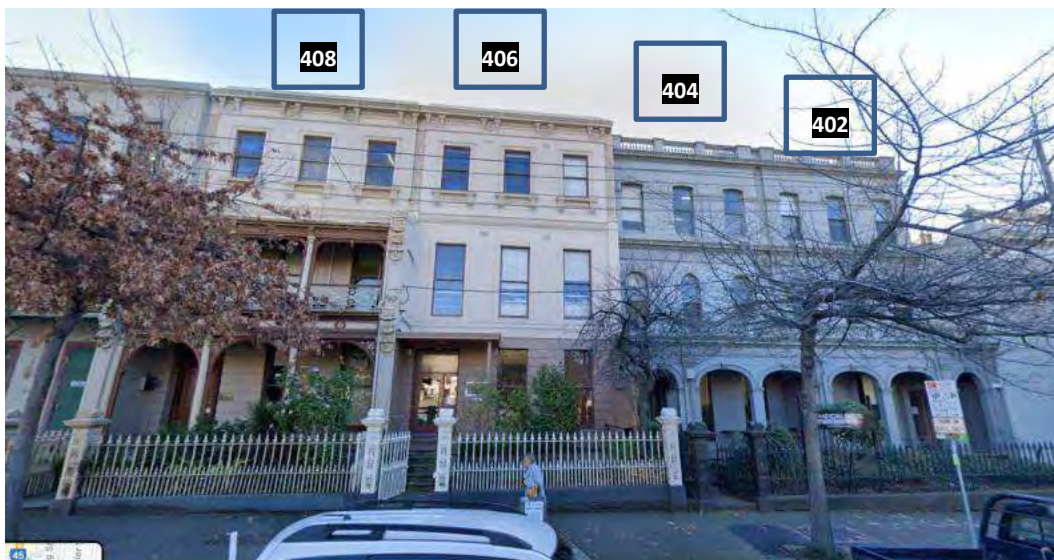
Figure 6 402-408 Albert Street, East Melbourne
