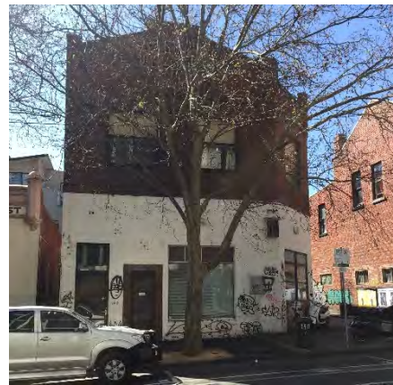
Figure 11 144-146 Queensberry Street, Carlton (HO807) Source: Lovell Chen
