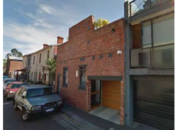
Figure 9 13-23 David Street, Carlton (HO1) Source: Streetview
