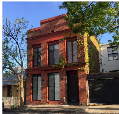
Figure 13 49 Owen Street, Carlton (HO1) Source: Lovell Chen
