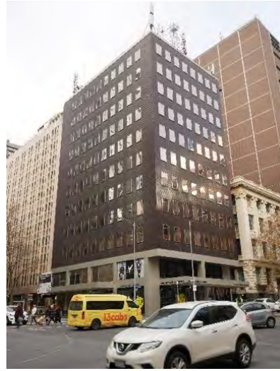
Former State Saving Bank of Victoria, 233-243 Queen Street (Godfrey & Spowers, Hughes Mewton and Lobb, 1967-68)
