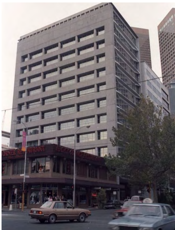
Figure 8. The building in 1984 (City of Melbourne Libraries online Heritage Collection, Reference no. Butler13724).
