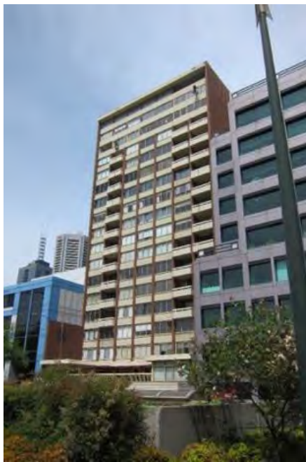
Park Tower, 199-207 Spring Street (Kurt Popper, 1969) (Interim HO1263)
