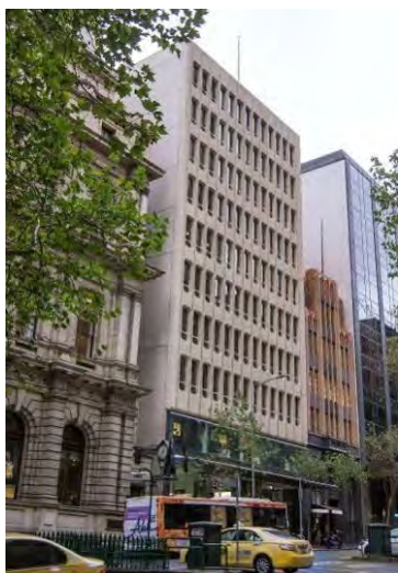
Former National Bank of Australasia Stock Exchange Branch, 85-91 Queen Street (Meldrum & Partners, 1973)
