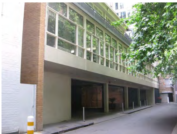
Figure 2. Lyceum Club, 2-18 Ridgway Place constructed 1959.
