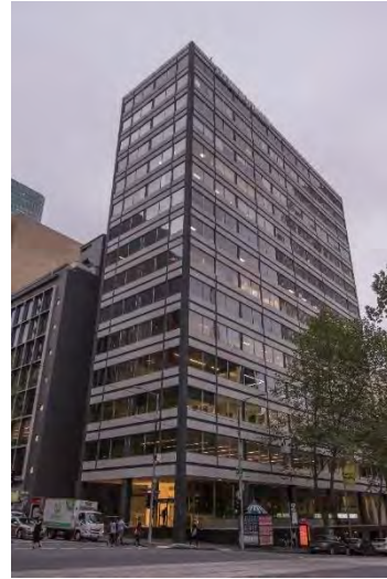
Former Sleigh Corner Building, 158-164 Queen Street (Bates Smart & McCutcheon, 1964)
