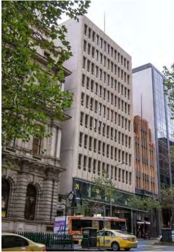
Former National Bank of Australasia Stock Exchange Branch, 85-91 Queen Street (Meldrum & Partners, 1973)
