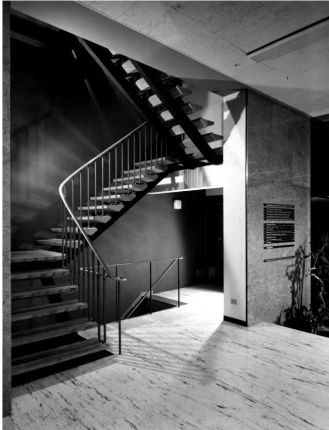
Figure 5. The foyer to building, photo dated 1961 (SLV, Wolfgang Sievers, photographer, Image H99.50/60).
