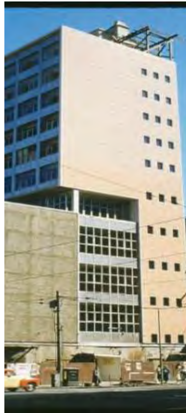
Figure 7. The construction phase. Photo probably dates to 1955-56 (SLV, Peter Wille, photographer, Image H91.244/3970).
