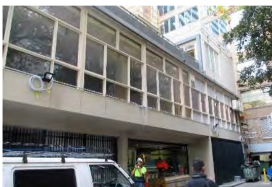
Figure 5. 2-18 Ridgeway Place, built in 1959. (Source: Context 2017)
