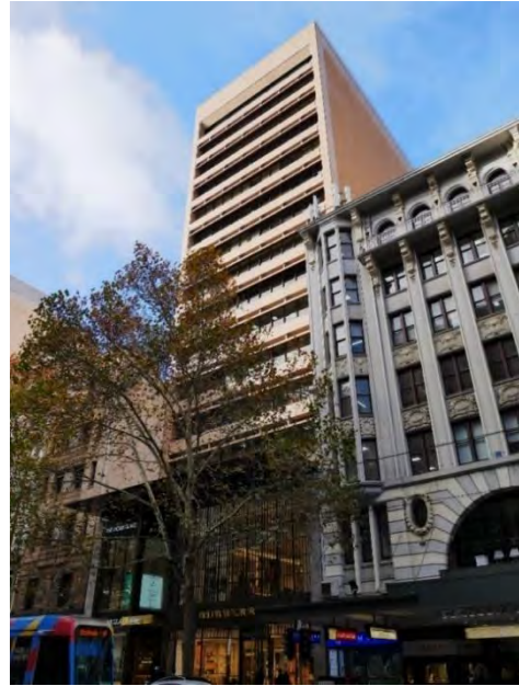
Former Commercial Banking Company of Sydney Building, 251-257 Collins Street, (Bates Smart & McCutcheon, 19741-73 included in HO502 The Block Precinct (fronting Collins Street) & HO506 (fronting Flinders Lane) (Non-contributory).
