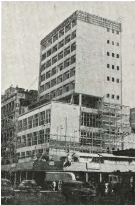
Figure 6. The construction phase, July 1955 ( Cross-Section , Jul 1955).
