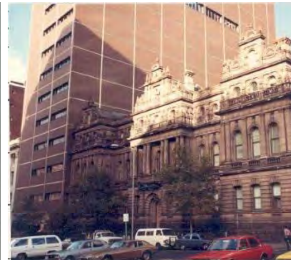
Figure 6. The subject building in 1985. (Source: Butler 1984: property key 105711)
