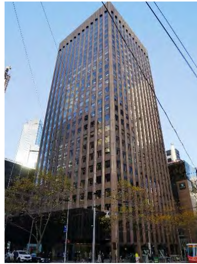
AMP Tower and St James Building Complex, 527-555 Bourke Street (Skidmore Owings & Merrill in association with Bates Smart & McCutcheon, 1965-69)
