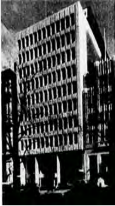
Figure 3. A 1998 photograph shows the building prior to its refurbishment in 2002, which saw the first floor extended to the building line and glazed. In the above image, the first floor is clearly recessed beneath the upper levels and the double height street level under-croft and colonnade is clearly intact. (Source: Age 16 September 1998:30)
