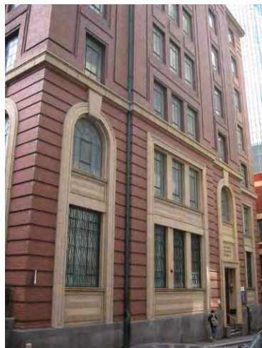
Figure 9. Telstra City West Exchange Building, 436 Little Bourke Street, Melbourne, built in 1937.
