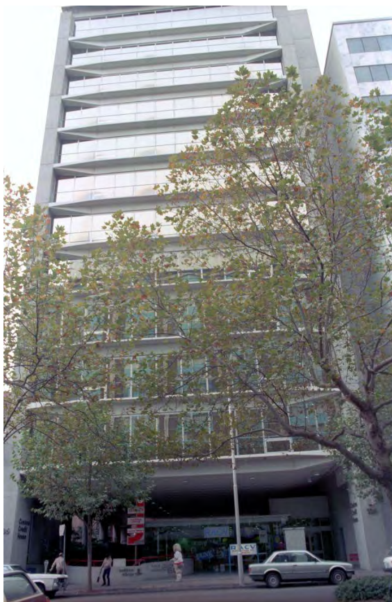
Figure 9. The ground and lower levels of the west elevation in 1984 (City of Melbourne Libraries online Heritage Collection, Reference no. Butler13723).
