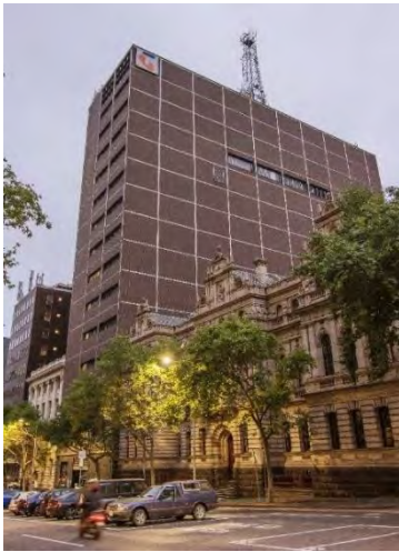
Lonsdale Exchange, 447-553 Lonsdale Street (Commonwealth Department of Works, 1969)
