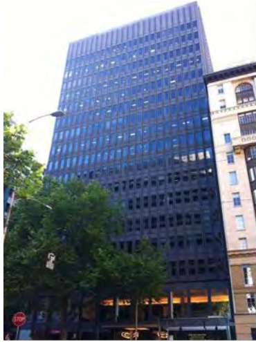
Royal Insurance Group Building, 430-442 Collins Street, (Yuncken Freeman, 1965) (Interim HO1010)
