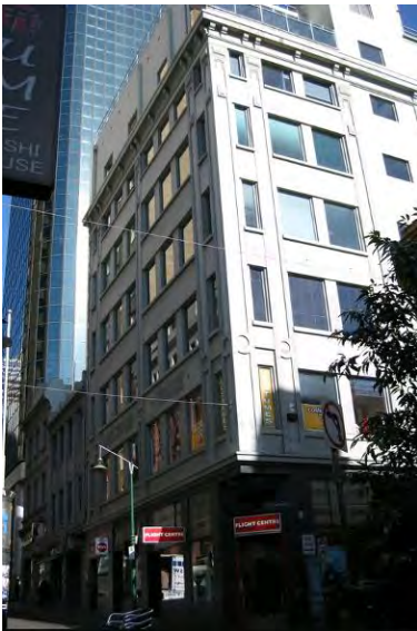
Figure 8. 386-392 Little Bourke Street, built in 1926.
