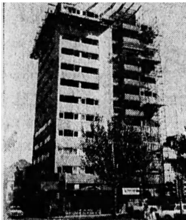
Figure 4. Image of the building under construction, published in May 1970 in a sales advertisement for the units ( Age , 2 May 1970:39).
