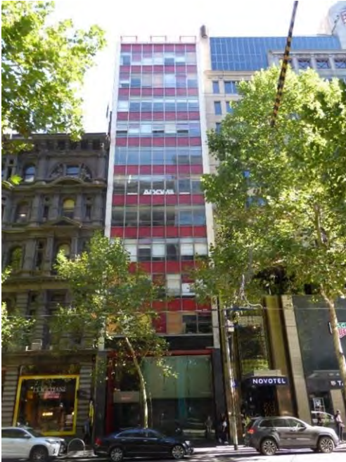
Former Allans Building, 276-278 Collins Street (Godfrey & Spowers, Hughes, Mewton & Lobb, 1956-57) included in HO502 The Block Precinct as a Contributory place.
