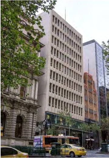
Former National Bank of Australasia Stock Exchange Branch, 85-91 Queen Street (Meldrum & Partners, 1973)
