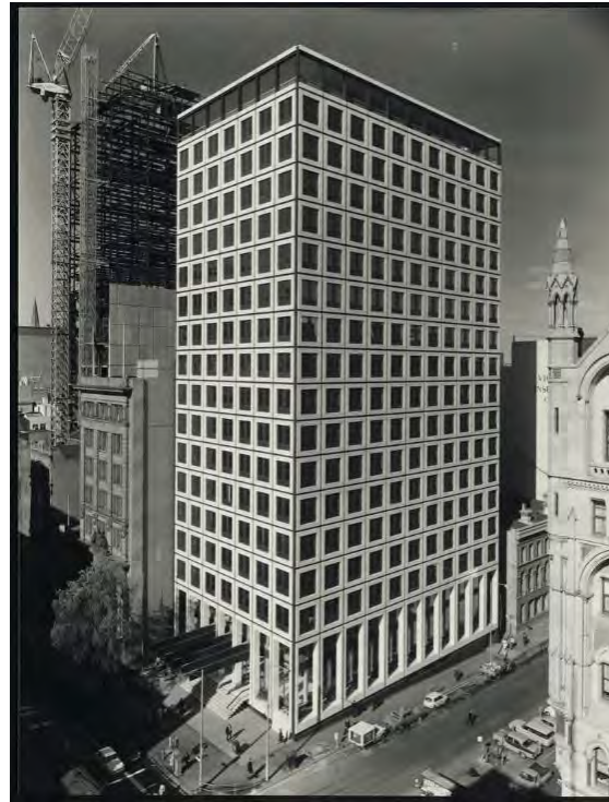
Figure 4. Photograph showing Legal & General House completed. (Source: Crothers 1967, SLV)
