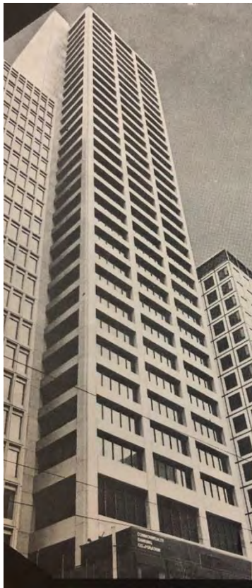
Figure 5. Illustration of the building published in the Nov/Dec 1974 issue of Architect , advertising reconstructed granite cladding by Melocco.
