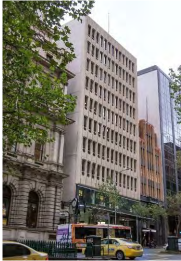
Former National Bank of Australasia Stock Exchange Branch, 85-91 Queen Street (Meldrum & Partners, 1973)
