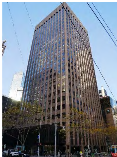
AMP Tower and St James Building Complex, 527-555 Bourke Street (Skidmore Owings & Merrill in association with Bates Smart & McCutcheon, 1965-69)
