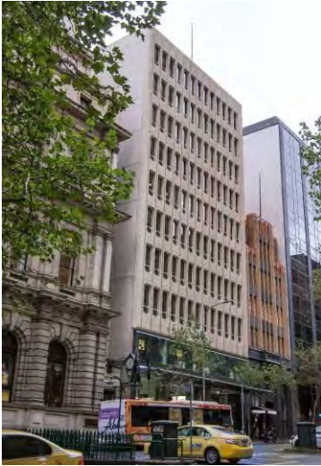
Former National Bank of Australasia Stock Exchange Branch, 85-91 Queen Street (Meldrum & Partners, 1973)
