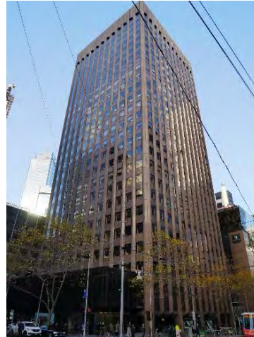
AMP Tower and St James Building Complex, 527-555 Bourke Street (Skidmore Owings & Merrill in association with Bates Smart & McCutcheon, 1965-69)
