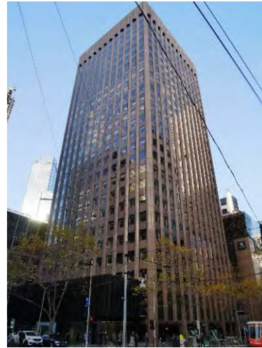
AMP Tower and St James Building Complex, 527-555 Bourke Street (Skidmore Owings & Merrill in association with Bates Smart & McCutcheon, 1965-69)
