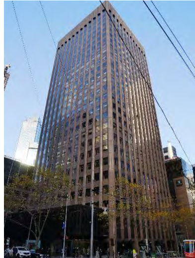
AMP Tower and St James Building Complex, 527-555 Bourke Street (Skidmore Owings & Merrill in association with Bates Smart & McCutcheon, 1965-69)
