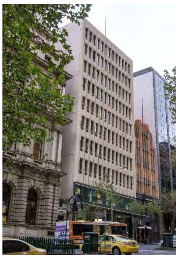
Former National Bank of Australasia Stock Exchange Branch, 85-91 Queen Street (Meldrum & Partners, 1973)
