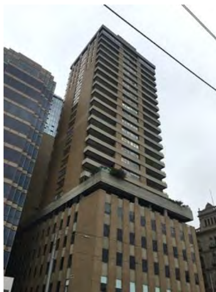
Treasury Gate, 93-101 Spring Street (Moore & Hammond, 1971) (Interim HO1262)
