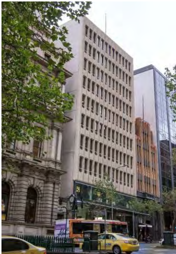
Former National Bank of Australasia Stock Exchange Branch, 85-91 Queen Street (Meldrum & Partners, 1973)
