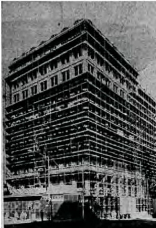
Figure 3. New Legal & General House under construction, 1966. (Source: Age 25 October 1966:13)
