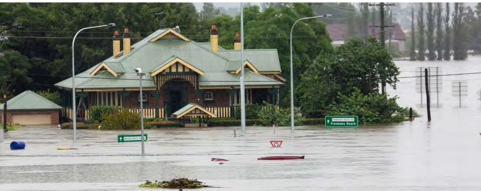
Figure 1: Roads and a new bridge submerged during a flood in Windsor, New South Wales, in 2021.
