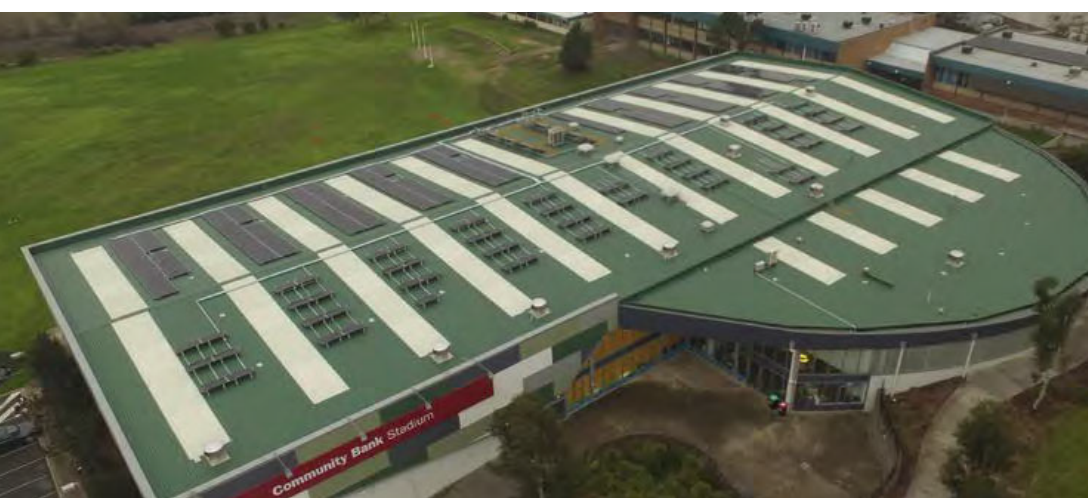
Figure 18: Nillumbik Shire Council's Community Stadium and Relief Centre in Victoria, featuring rooftop solar, a battery system and an electric vehicle charging station.
