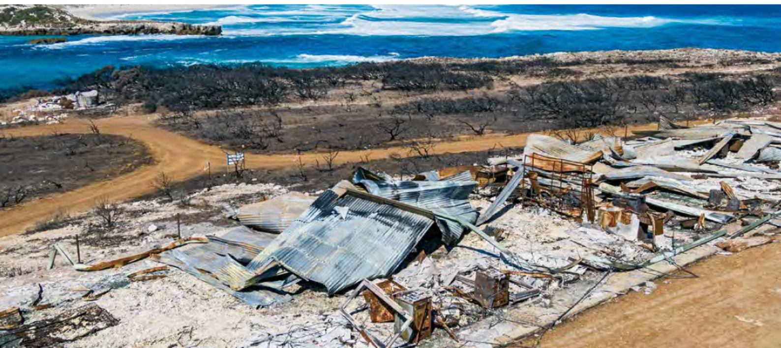
Figure 9: Holiday resort villas on Kangaroo island, South Australia destroyed by 2020 bushfires.
