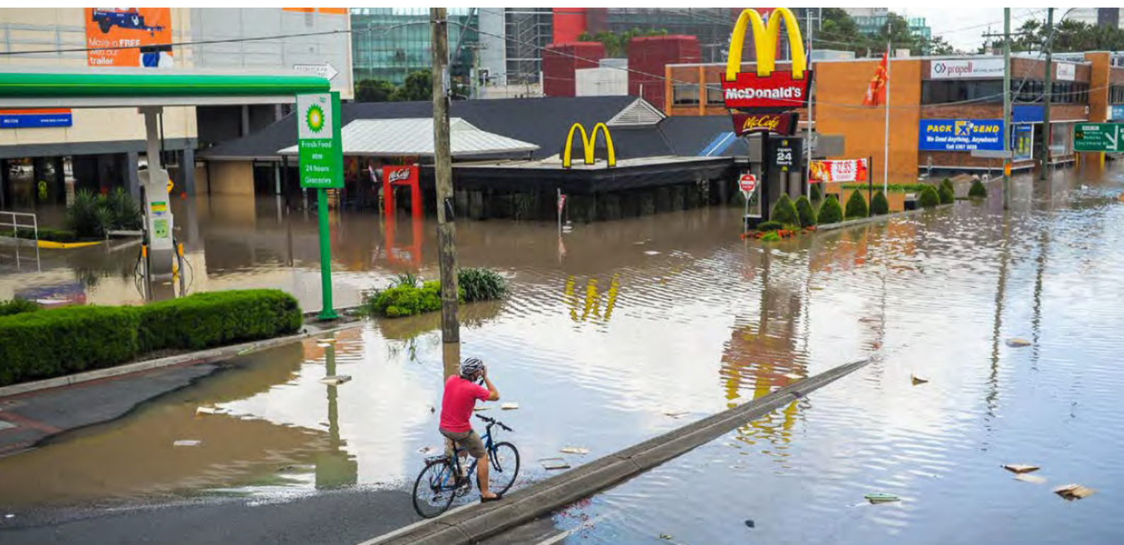
Figure 21: Damage from 2011 floods in Brisbane, Queensland.
