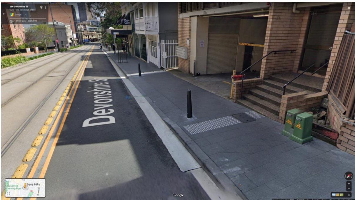
Example of continuous footpath treatment at a driveway in the City of Sydney
