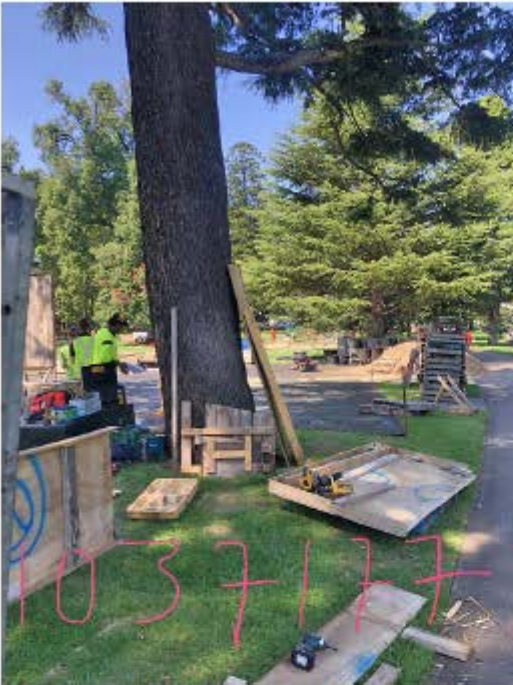
Photo 4: A view of a site where minor items were inappropriately stored near and against a tree (incident 4).
