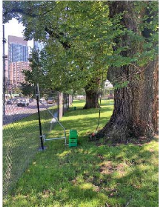
Photo 3: A view of the amended fence line treatment more in line with both the project arborist guidance and the TPP.
